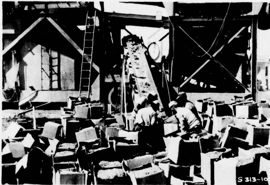
Figure 3-4. Introduction of fibers during batching of materials for fibrous concrete
