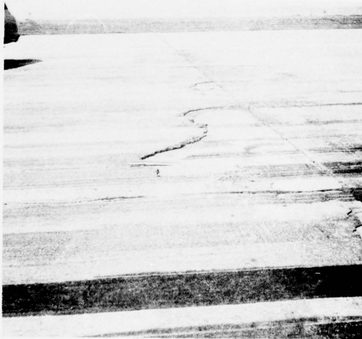
Photo 2. Raveling of feathered edge of AC at sta 165+03 of NW-SE runway
