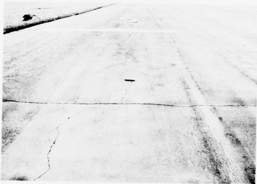
Photo 5. Taxiway T shoulder pavement
