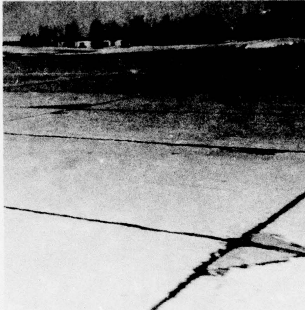
Photo 5. Condition of ADC operational apron
