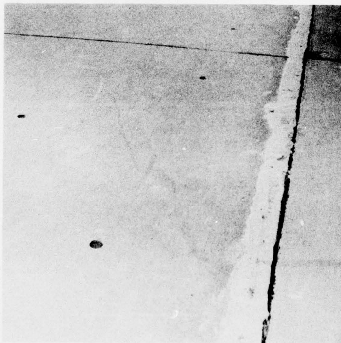
Photo 2. Epoxy patch and grouted drill holes
