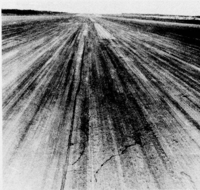
Photo 2. General view of runway near SE end of AC pavement
