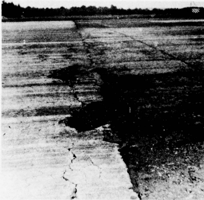
Photo 3. Pavement condition at junction of PCC and AC at SE end of runway
