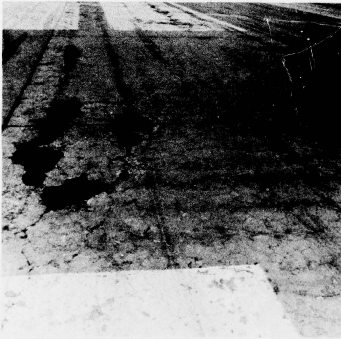
Photo 4. AC surface patches on PCC pavement at SE end of runway
