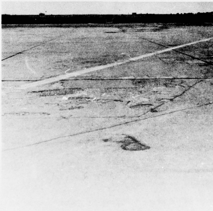
Photo 6. Sealing of slabs in north warm-up apron
