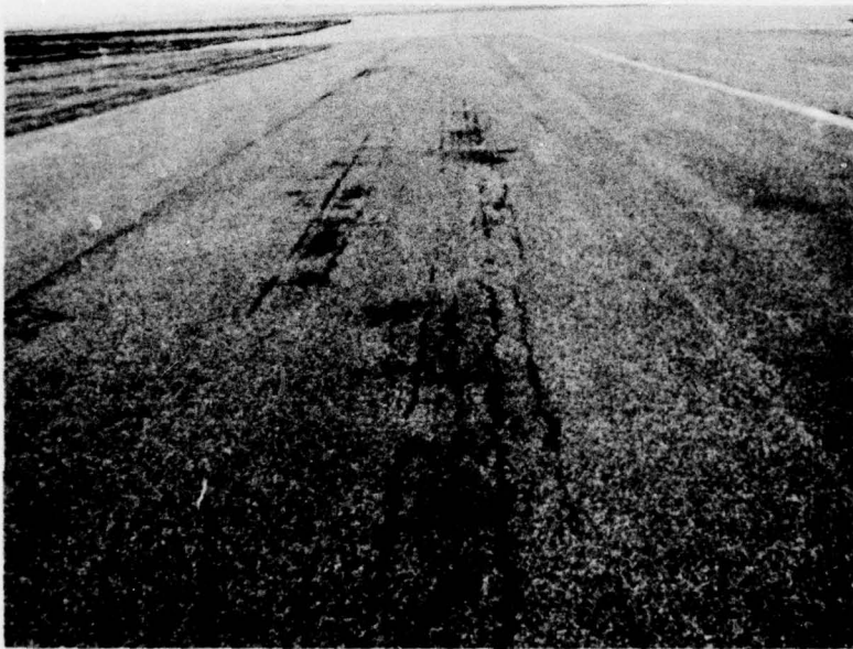
Photo 4. Typical condition of taxiway 4
