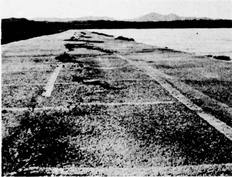
Photo 5. Showing of shoulder pavement along south end of parking apron
