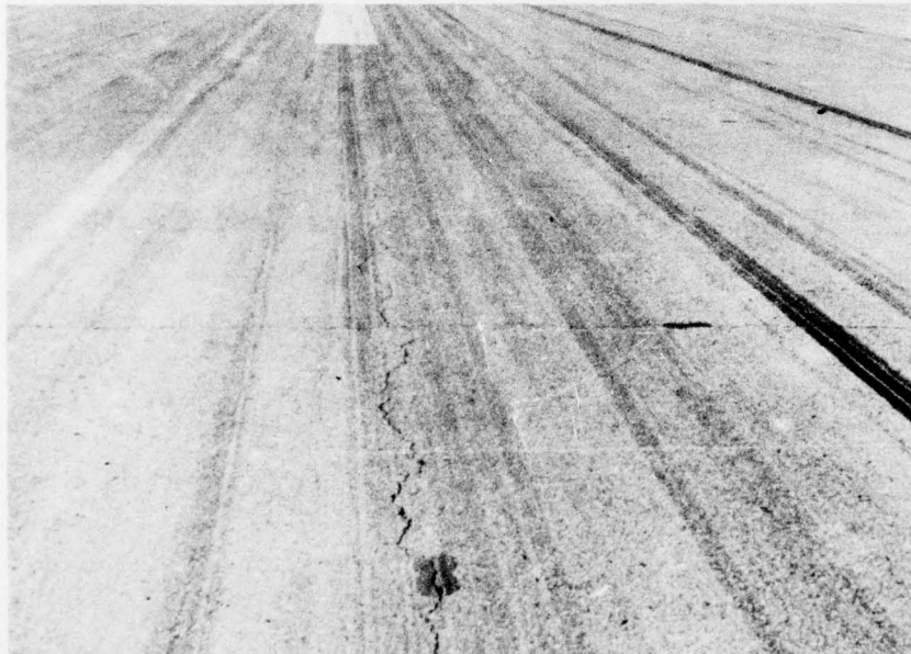
Photo 2. General view of runway looking south from sta 60+00
