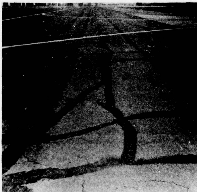
Photo 8. View of shoulder of taxiway S without slurry seal
