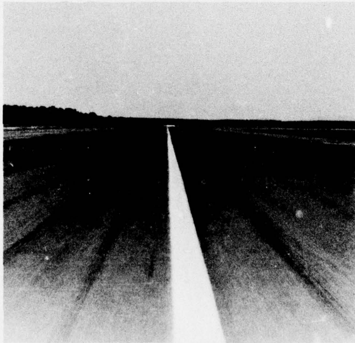
Photo 10. Typical view of NE end taxiway G opposite calibration hardstand
