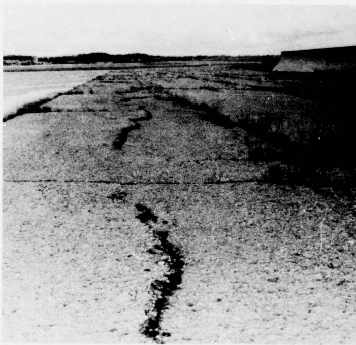
Photo 6. Shoving of shoulder pavement along heavy-load operational apron extension
