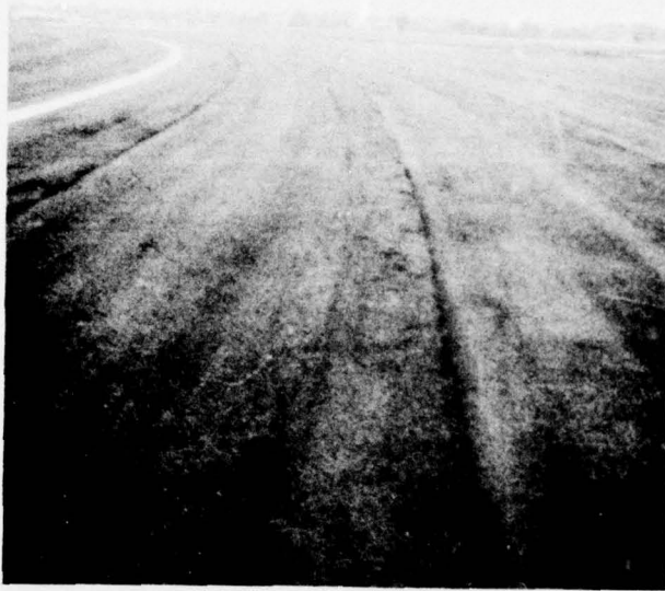
Photo 9. Paving lane joints in taxiway 10 and warm-up apron 1
