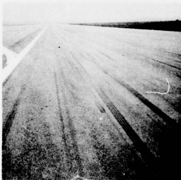
Photo 8. Good condition of taxiway 21 at intersection with taxiway 8
