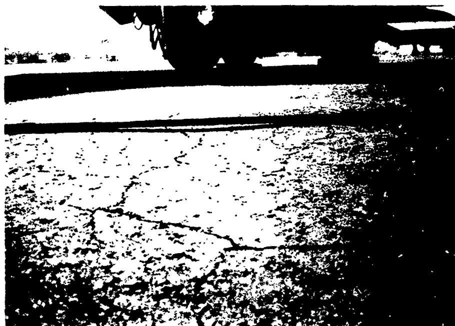
Photo 8. Ruts up to 1 in. deep in taxiway area of MacDill (1971) pavement
