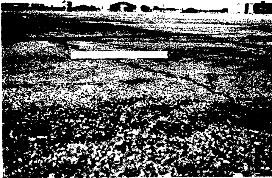
Photo 2. Unevenness on surface of Homestead (1955) pavement from cracking
