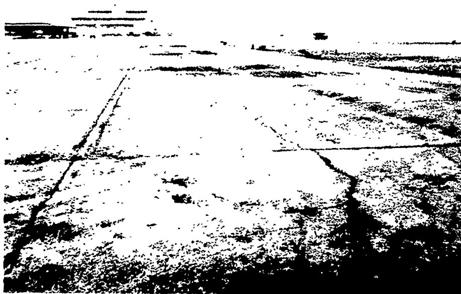
Photo 40. General deterioration of Wright-Patterson (1966) pavement from cracking and fuel spillage
