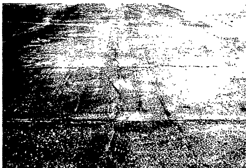
Photo 28. Reflection cracks in asphalt in foreground continuing through tar-rubber area where roofing felt was used in Mountain Home (1968) pavement
