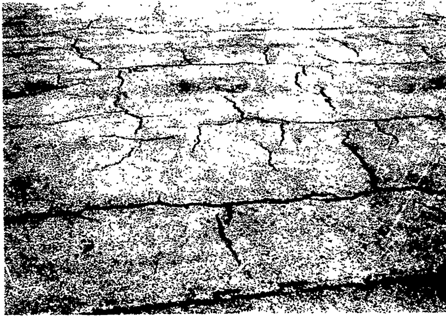
Photo 1. Block cracking in Homestead (1955) pavement
