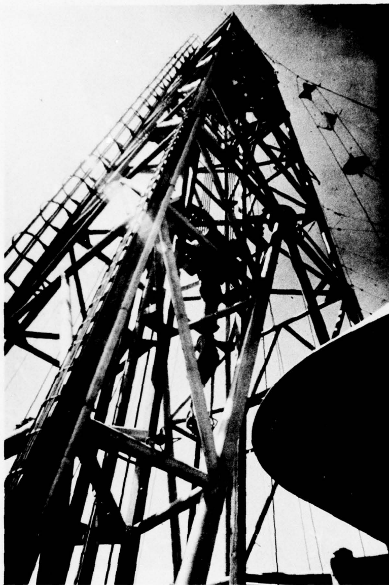
The Drill Pipe String is Raised into the Derrick by the Multi-ton Coupling.
