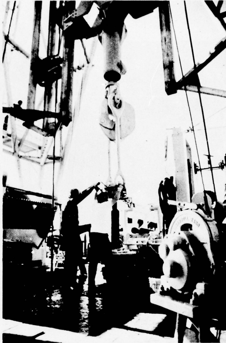
The Deck Crew Stands by for Orders from Search Central Adding to or Reducing the Length of the Pipe String.
