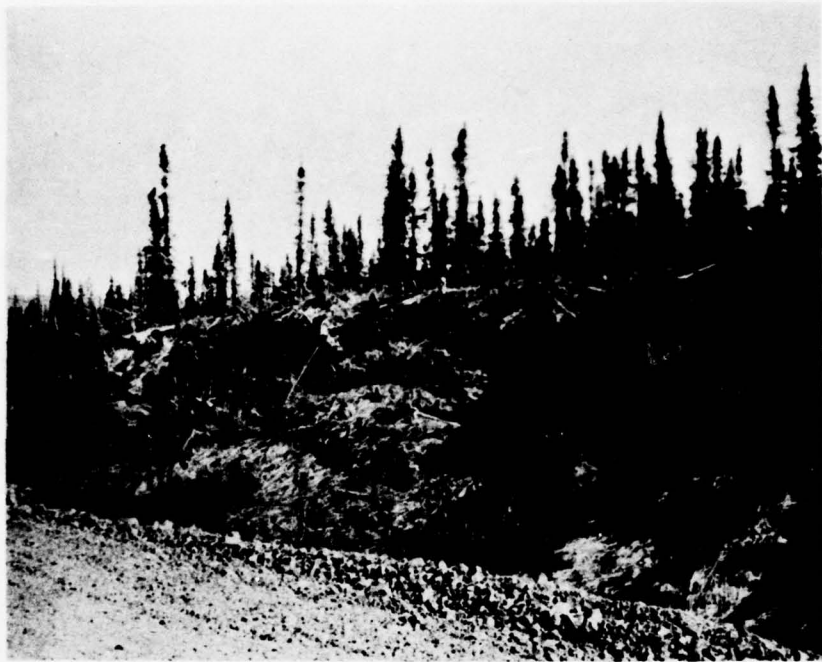
80. Center portion of slope, Mile 22.9 Rt, 17 August 1971.
