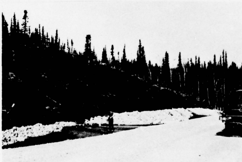
37. Receding backslope and stabilized ditch sediments, Mile 19.6 Lf, 23 May 1971.
