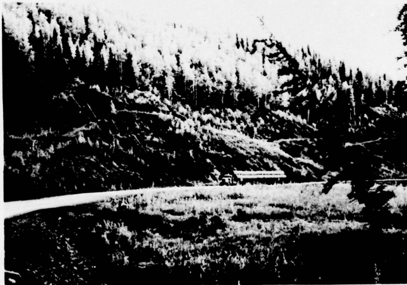
103. Overall view of backslope, Mile 33.3 Rt, 14 September 1975.
