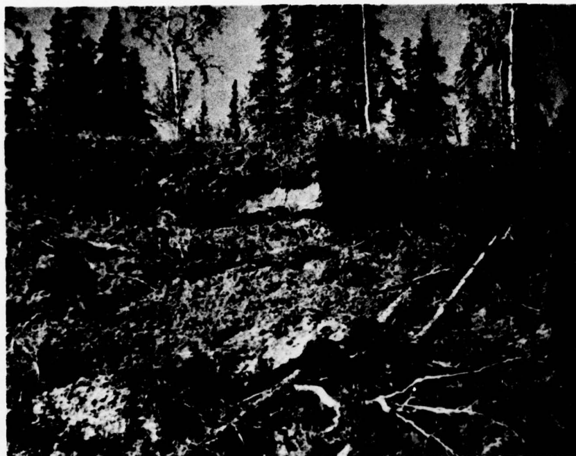
60. Untidy appearance and continued thawing of backslope, Mile 20.25 Lf, 17 August 1971.
