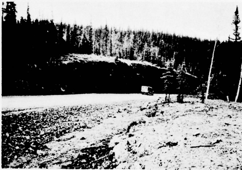
56. Ice face with overhanging mat and clearing atop backslope, Mile 20.25 Lf, 26 June 1970.
