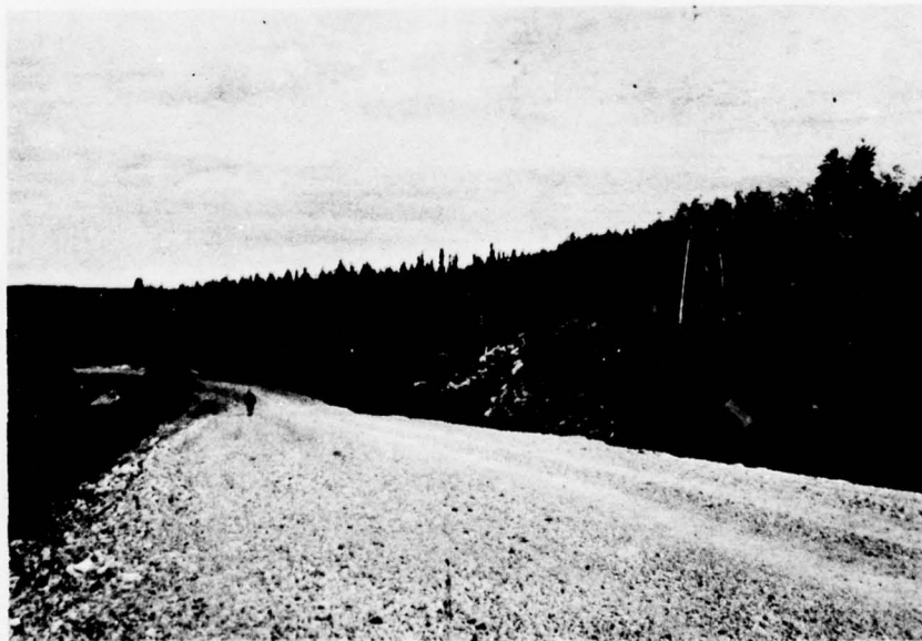
29. Overall view of deep cut, Mile 9.85 Rt, 17 August 1971.
