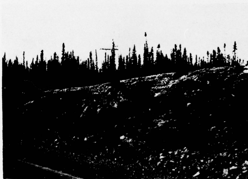
87. Overall view of backslope, Mile 23.2 Lf, 23 June 1972.
