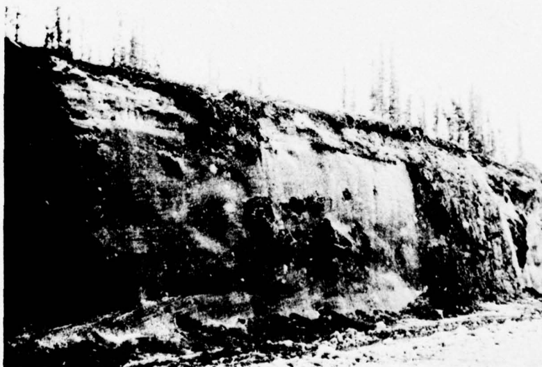
83. Massive ice in frozen backslope, Mile 23.2 Lf, 23 April 1970.
