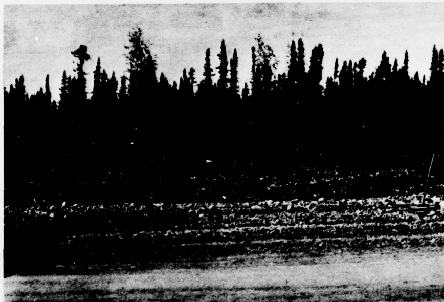
105. Left embankment slope, Mile 16.3, 27 June 1970.
