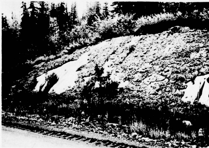
53. Insulated backslope, Mile 19.9 Lf, 14 September 1975.
