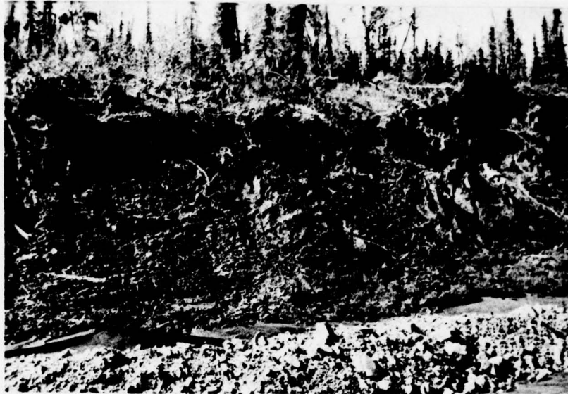
36. Mud flow on thawing backslope, Mile 19.6 Lf, 11 August 1970.
