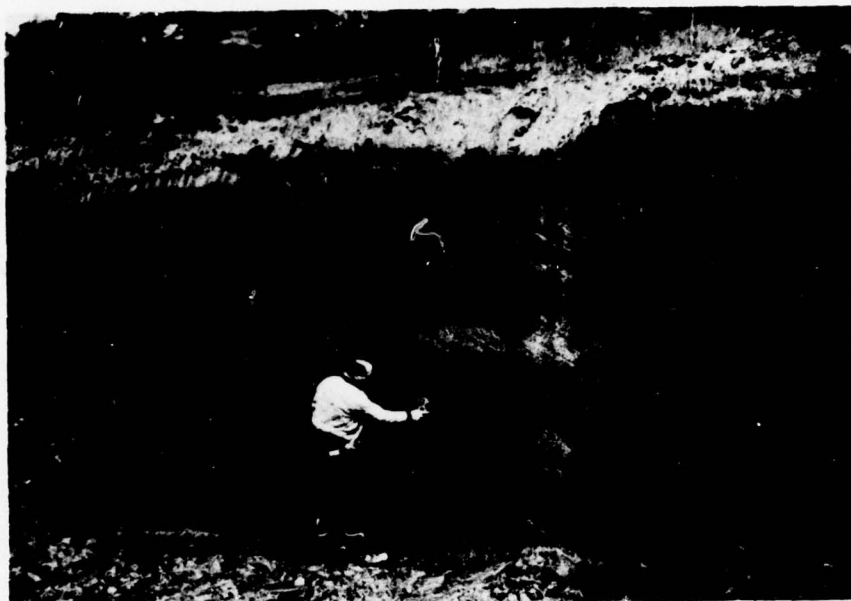
76. Massive ice in frozen backslope, Mile 22.9 Rt, 23 April 1970.
