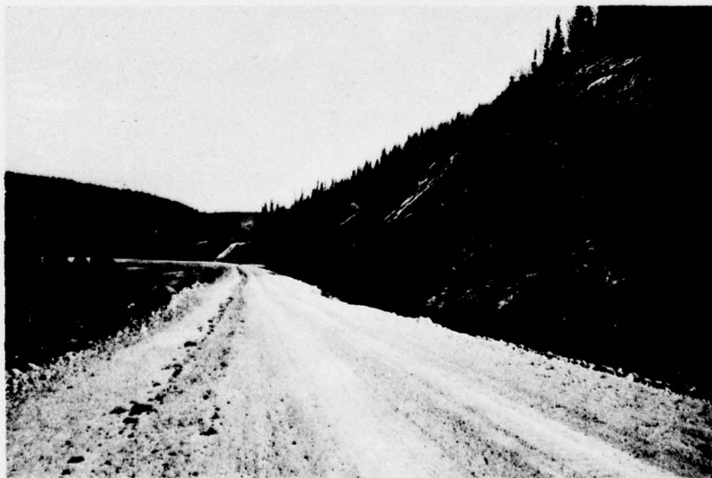
97. Benched slope, Mile 33.3 Rt, 28 May 1971.
