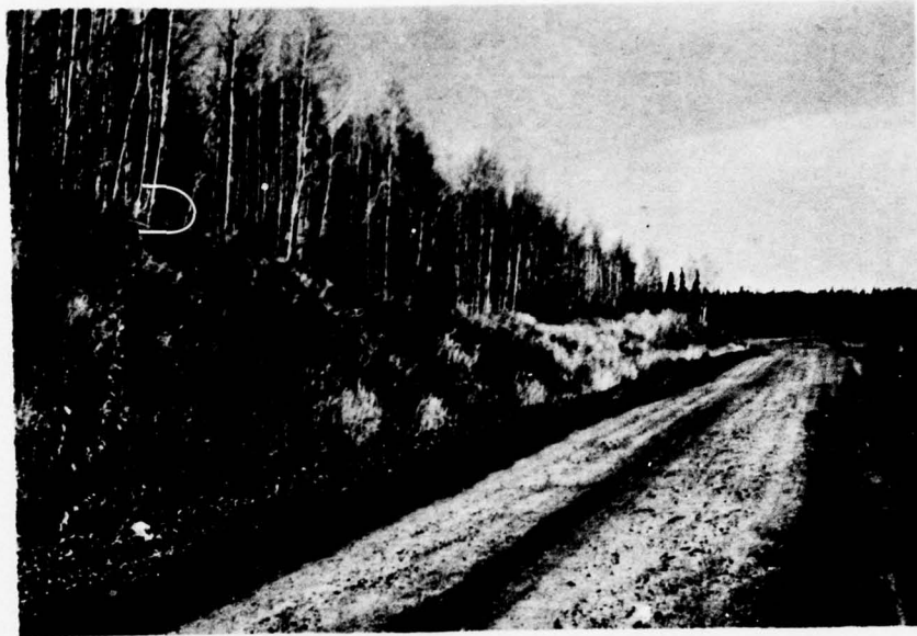
18. Southern end of backslope, Mile 4.5 Rt, 27 September 1974.
