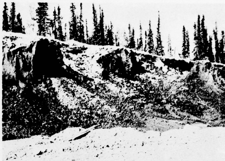
84. Center portion of slope showing fibrous insulation on cleared top of backslope, Mile 23.2 Lf, 11 August 1970.
