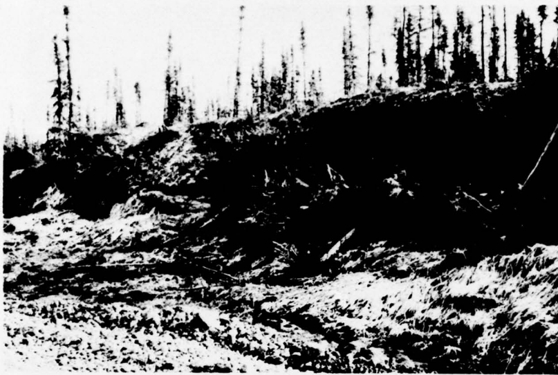
78. Center portion of slope, Mile 22.9 Rt, 28 May 1971.
