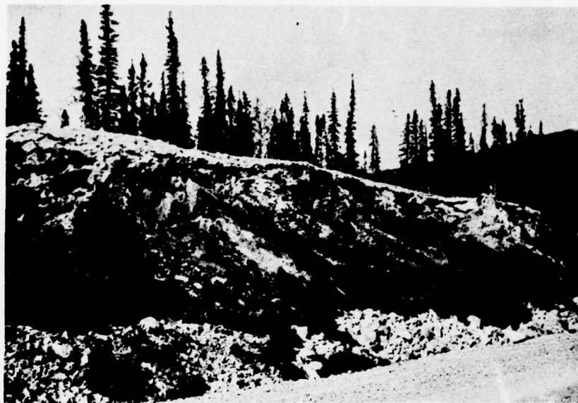
86. View of slope showing grass growth and continued slumping, Mile 23.2 Lf, 17 August 1971.
