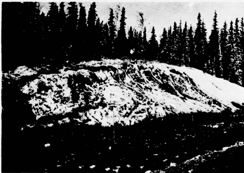
51. Insulation covering backslope, Mile 19.9 Lf, 27 September 1974.
