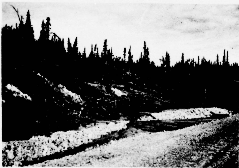
41. Overall view of slope showing toppling spruce trees, Mile 19.6 Lf, 23 June 1972.
