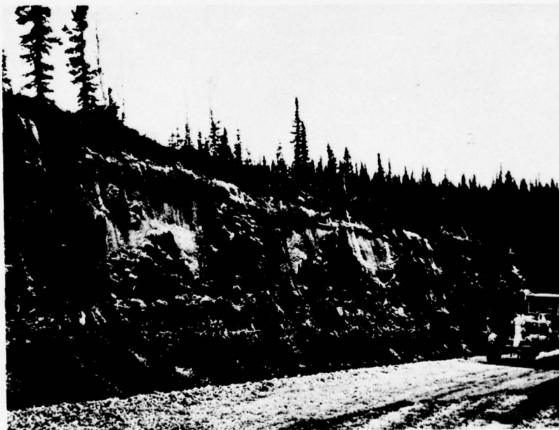
55. Frozen nearly-vertical backslope with large ice masses, Mile 20.25 Lf, 23 April 1970.
