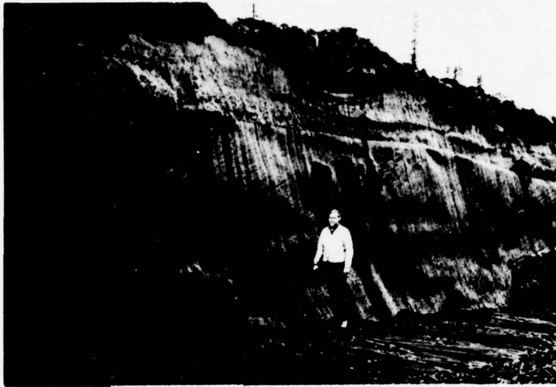
68. Massive ice in frozen backslope, Mile 22.9 Lf, 23 April 1970.
