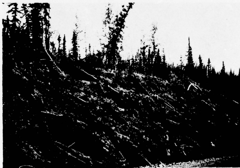
61. Overall view of slope, Mile 20.25, 23 June 1972.
