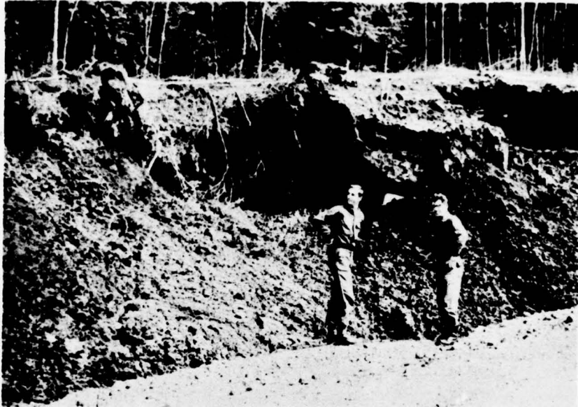
10. Organic mat overhanging part of thawing backslope, 26 June 1970.
