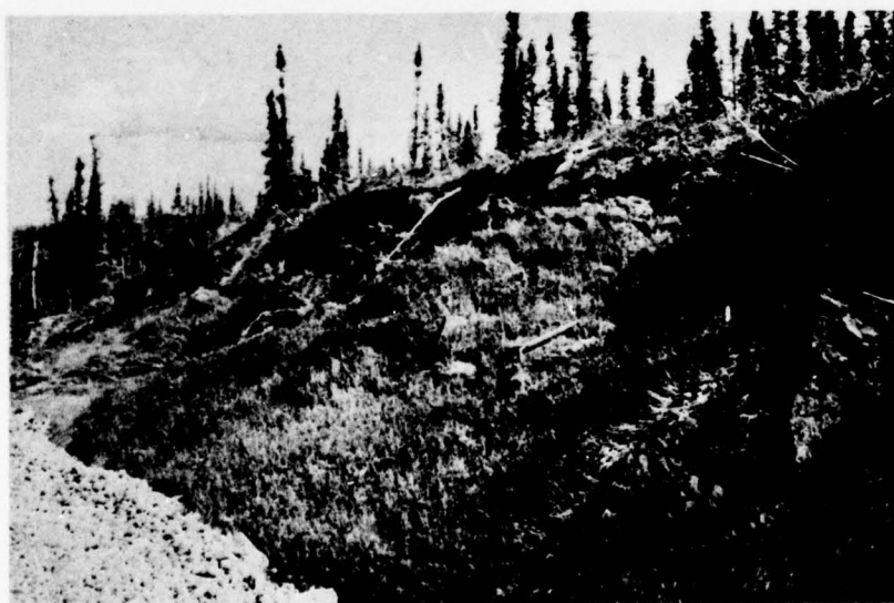
77. Parts of backslope stabilized and other sections receding, Mile 22.9 Rt, 11 August 1970.
