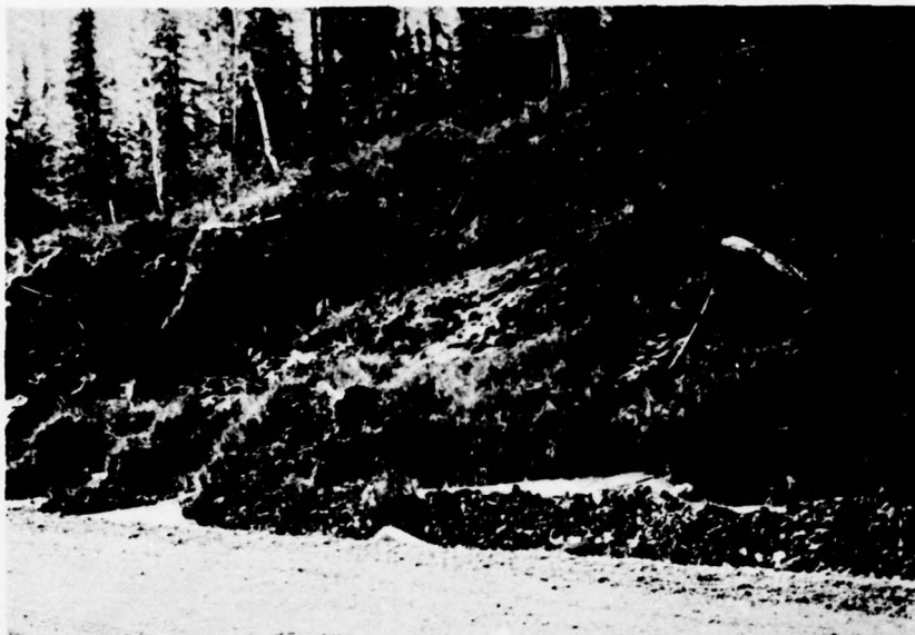
46. Seeded backslope, overhanging mat and broken rock revetment, Mile 19.9 Lf, September 1970.
