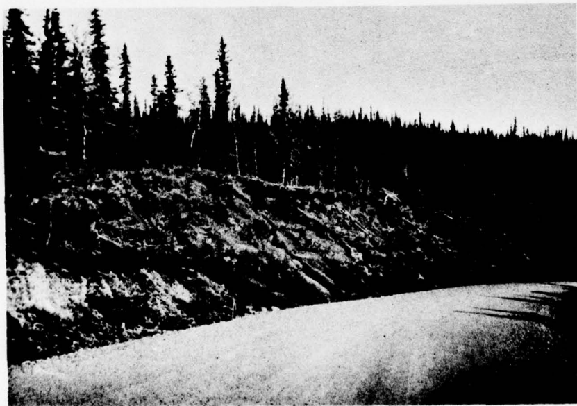
59. Overall view of slope, Mile 20.25 Lf, 17 August 1971.
