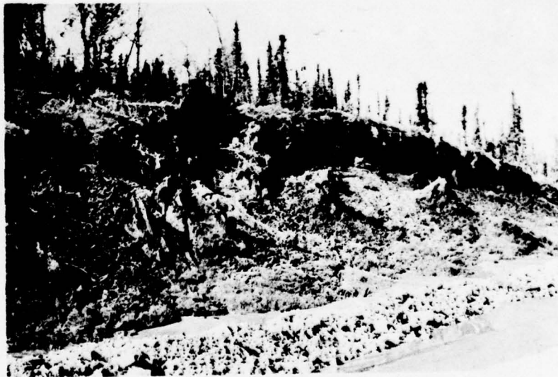
35. Thawing slope receding into limit of clearing, Mile 19.6 Lf, 11 August 1970.
