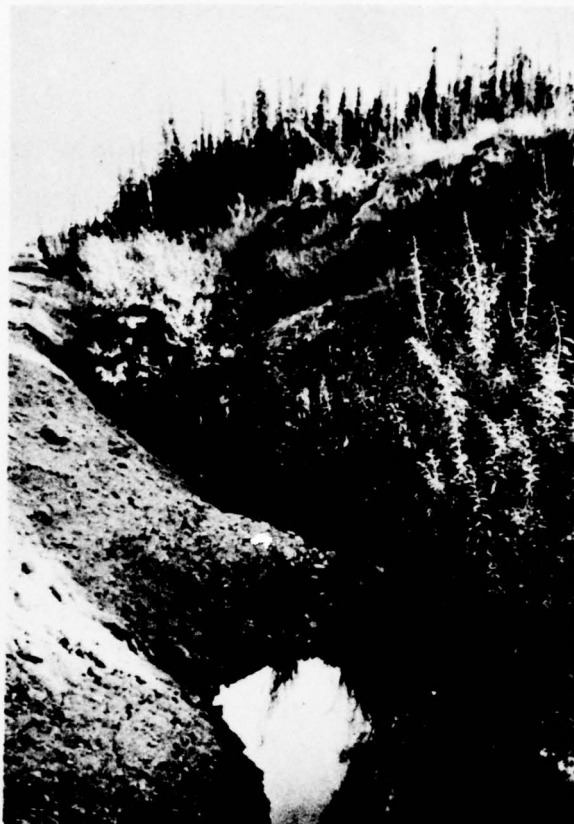
8. Thaw subsidence in ditch at Mile 23.2 Lf.
