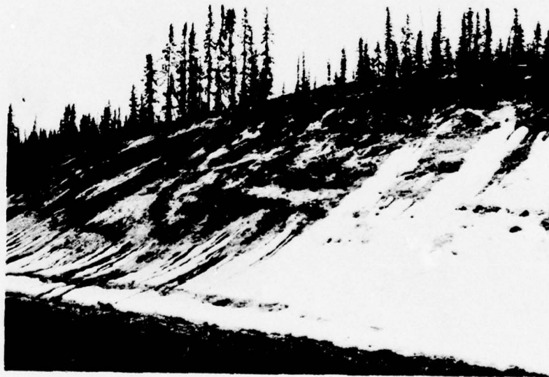
31. Frozen, partially snow-covered 1:1 backslope, Mile 19.6 Lf, 23 April 1970.
