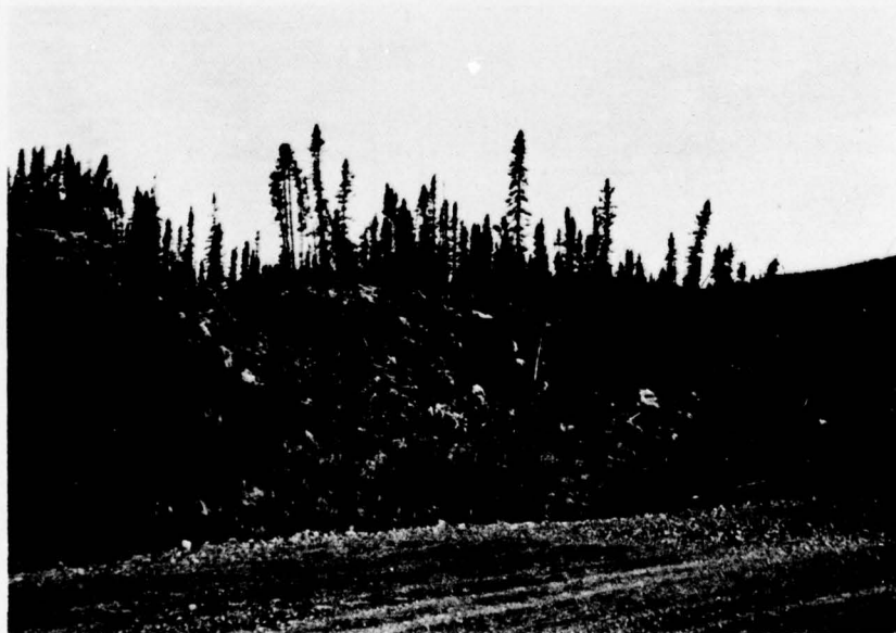
73. Continued instability of backslope, Mile 22.9 Lf, 23 June 1972.
