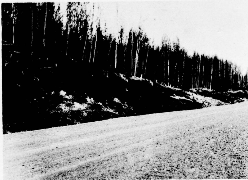
13. Southern end of receding and seeded backslope, Mile 4.5 Rt, 27 May 1971.
