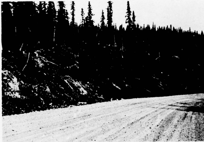
58. Overall view of slope, Mile 20.25 Lf, 28 May 1971.
