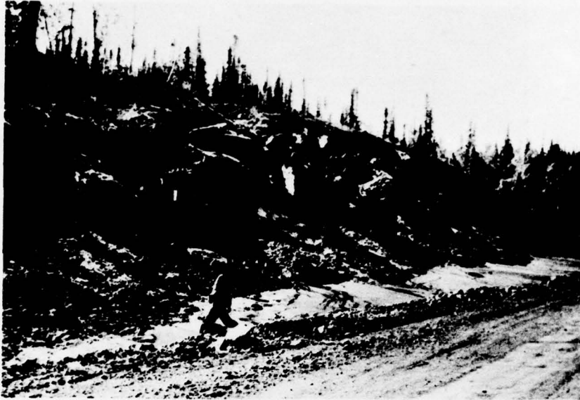
32. Thawing backslope, Mile 19.6 Lf, 26 June 1970.
