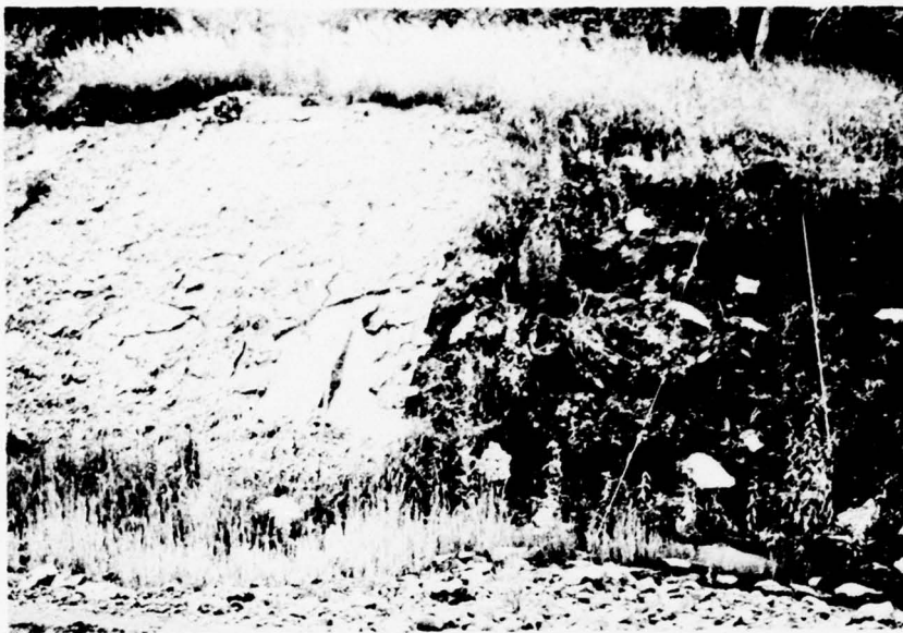
54. Insulated and uninsulated portions of backslope, Mile 19.9 Lf, 14 September 1975.
