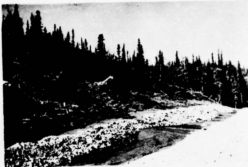
34. Seeded backslope and broken rock revetment, Mile 19.6 Lf, 11 August 1970.
