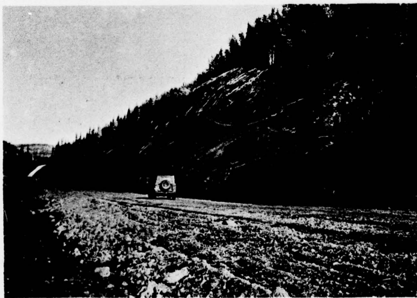
93. Overall view of backslopes, Mile 33.1 and 33.3 Rt, September 1970.
