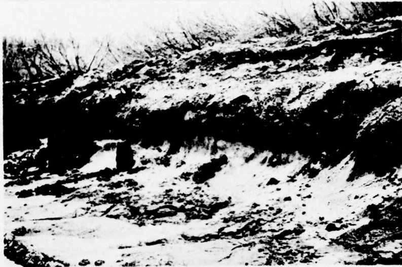
22. Massive ice in shallow cut, Mile 9.85 Rt, 23 April 1970.
