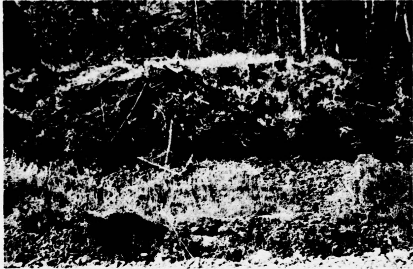
48. Part of backslope appearing fairly stable, Mile 19.9 Lf, 17 August 1971.
