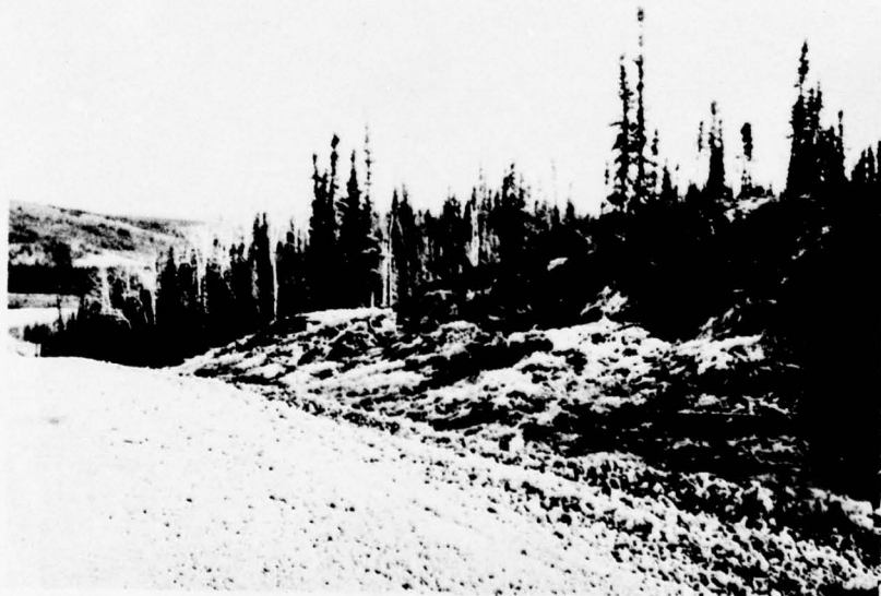
79. Northern portion of slope, Mile 22.9 Rt, 23 June 1972.
