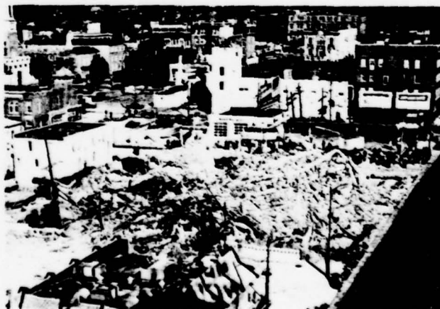
FIGURE 19. THE FORT WAYNE, INDIANA, KEENAN HOTEL EXPLOSIVE DEMOLITION PROJECT
