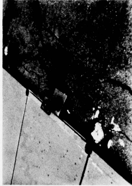
Photo 6. Mat movement at east edge of runway, Sta 10+00
