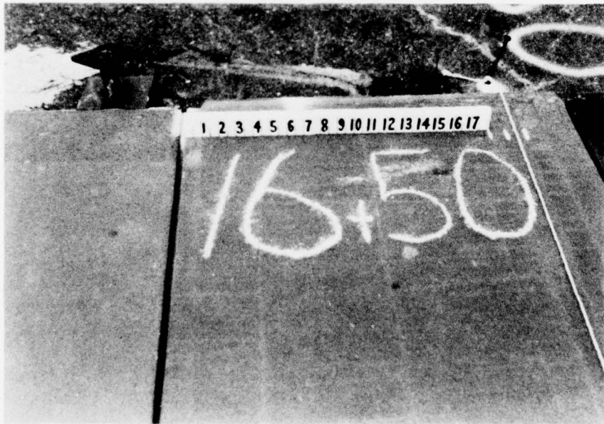
b. Mat moved 19-3/4 in. along west edge Runway moved south (left) after 300 sorties
