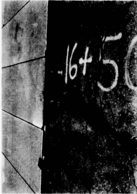
Photo 10. Mat movement, east edge of runway, Sta 16+50
