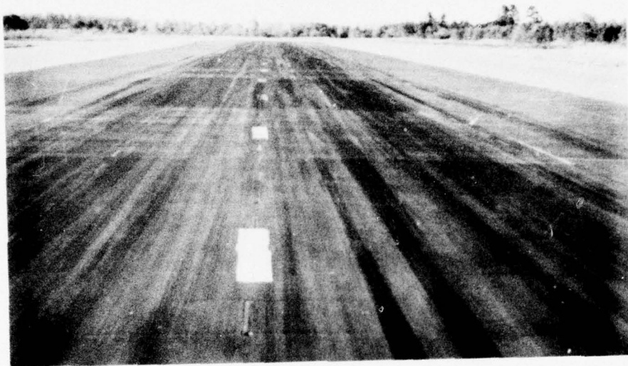
View looking north at sta 5+00 showing skid marks in touchdown area
