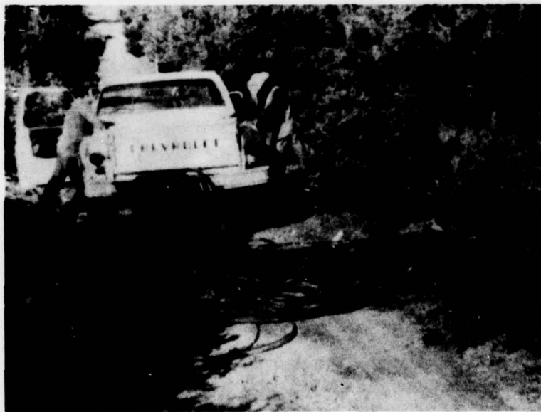
Figure 44. Spiral-4 cable attached to truck prior to dragging to cleared area from brush entanglement
