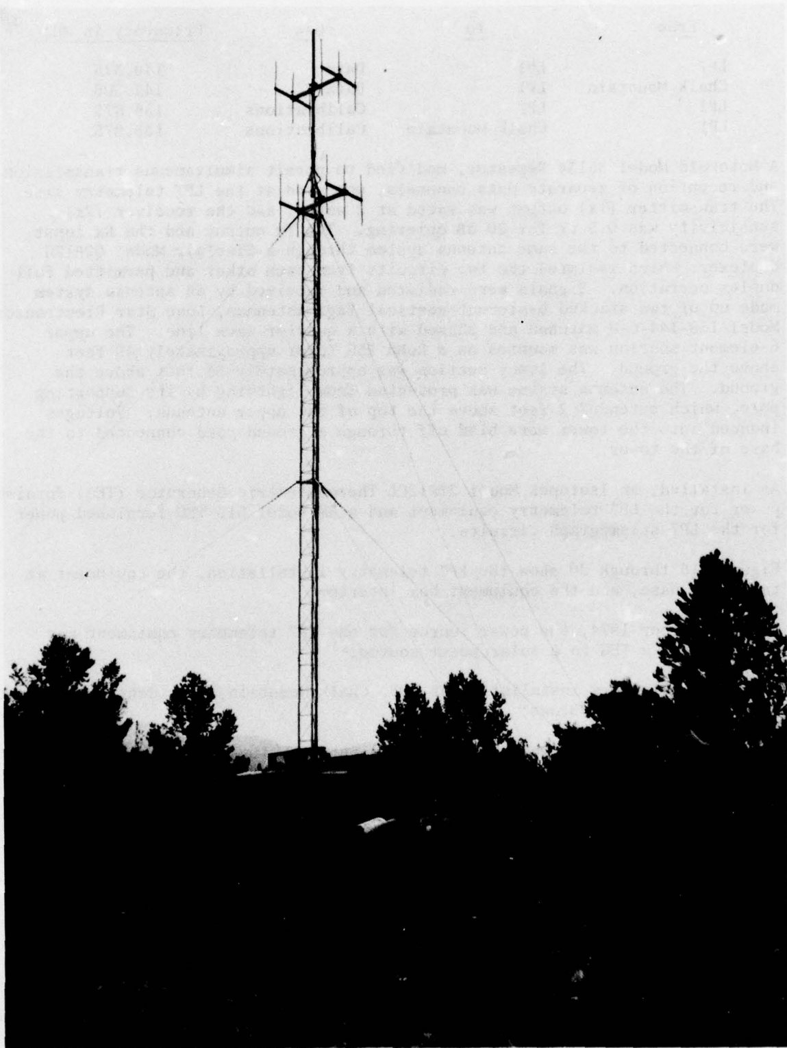
Figure 18. Radio telemetry installation near LP7
