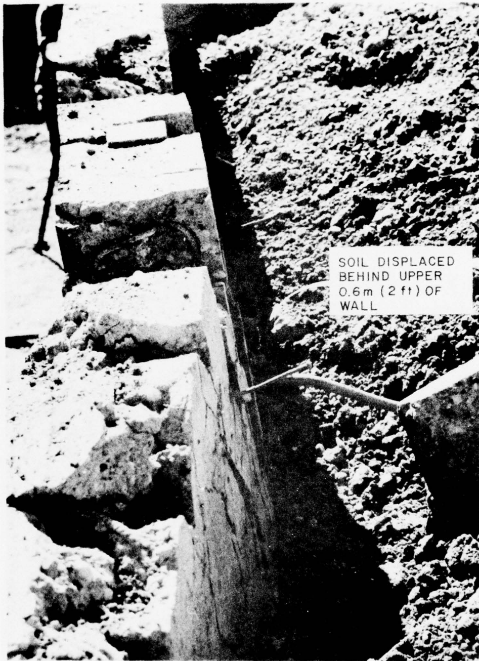
Fig 20 Soil displacement at rear of Wall No. 1, Test No. 3
