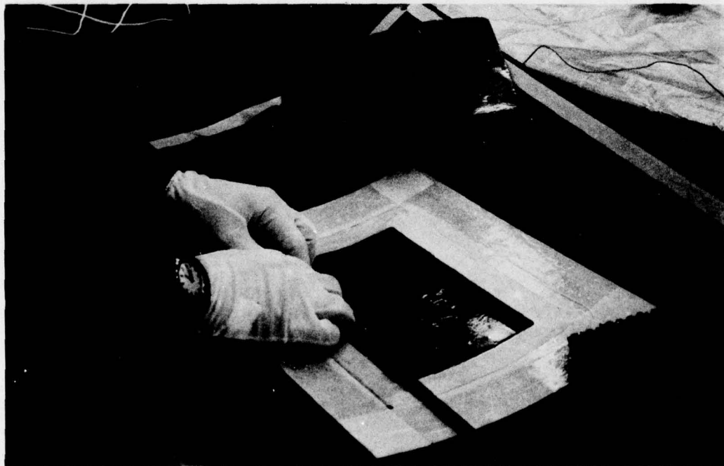
Figure 43.—Installation of the Core Splice Adhesive
