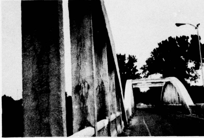
a. Overall view
