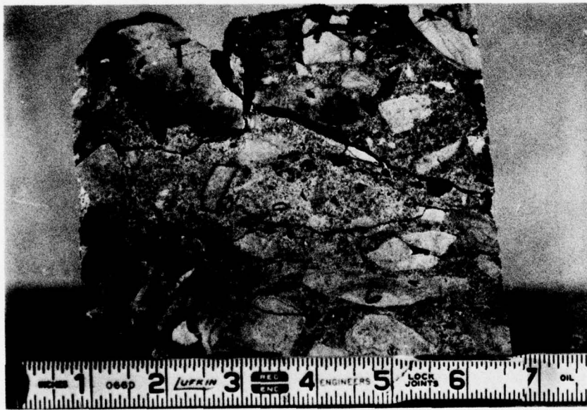
b. Section of core 6 from the North Abutment prepared as above. The surface shows several limestone coarse aggregate particles with reaction rims (upper, lower areas). These were involved in an alkali-carbonate rock reaction.
