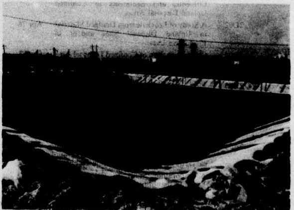
One of four 24 x 24 m test pits with different underdrain configurations used to evaluate the effectiveness of underdrains to dewater fine-grained dredged material ( Work Unit 5A15 )
