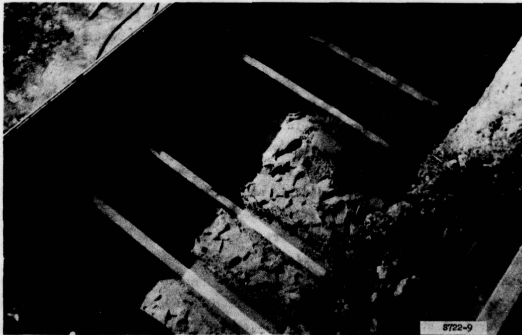
Figure 19. Reinforcing strips spread evenly on surface of sand
