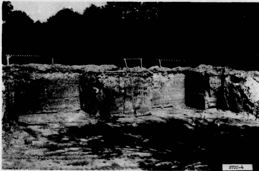
Figure 17. Test pits after walls were smoothed by front-end loader
