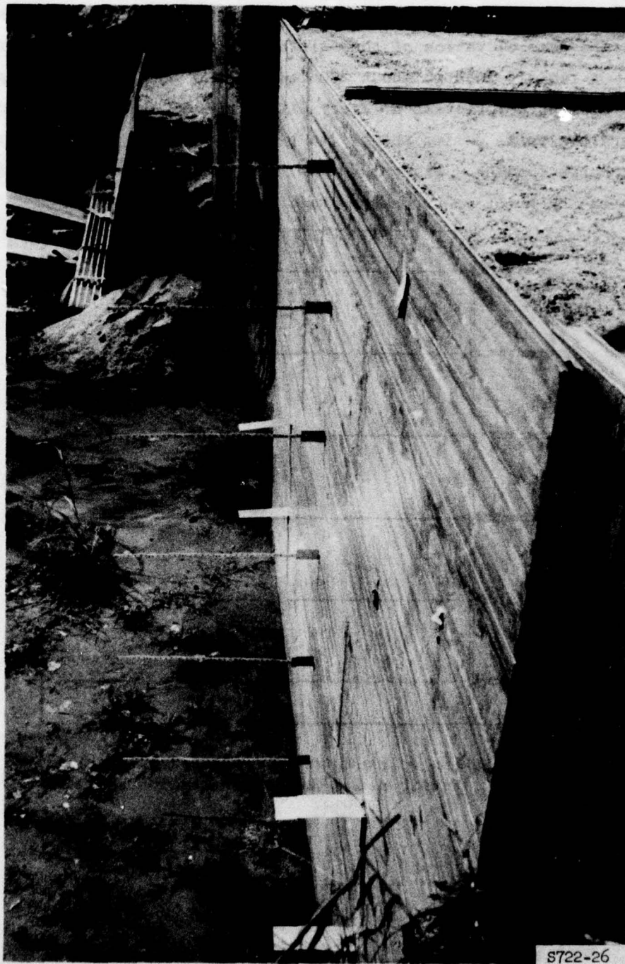
Figure 27. Reinforced earth retaining wall prior to surcharge loading
