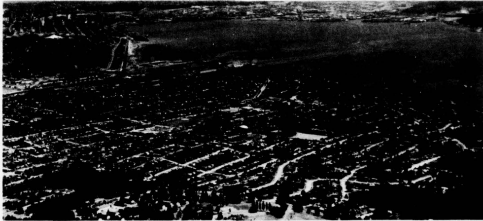
Urban land, an increasing important use of the land resources of the C-NP Region (Port of Seattle)
