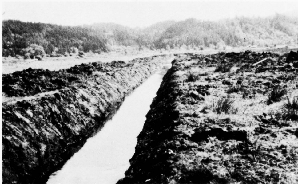
Main outlet ditch for tile drains. (SCS 0-1030-5)
