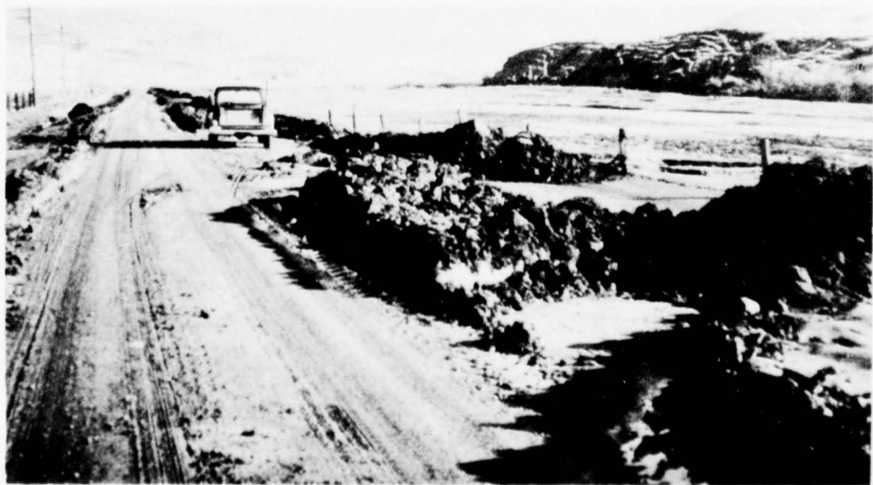
Sedimentation removal from roads and road ditches is expensive, causes hazards, and reduces or restricts essential transportation. (SCS 0-1738-11)
