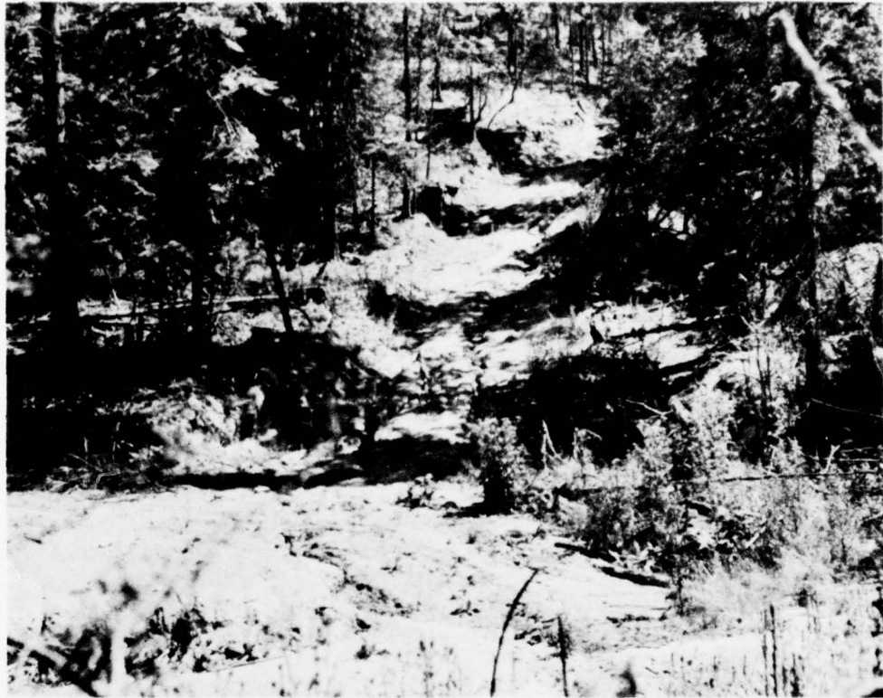
Lack of cross-drainage or revegetation resulted in gullies on an abandoned tractor road. (Forest Service)
