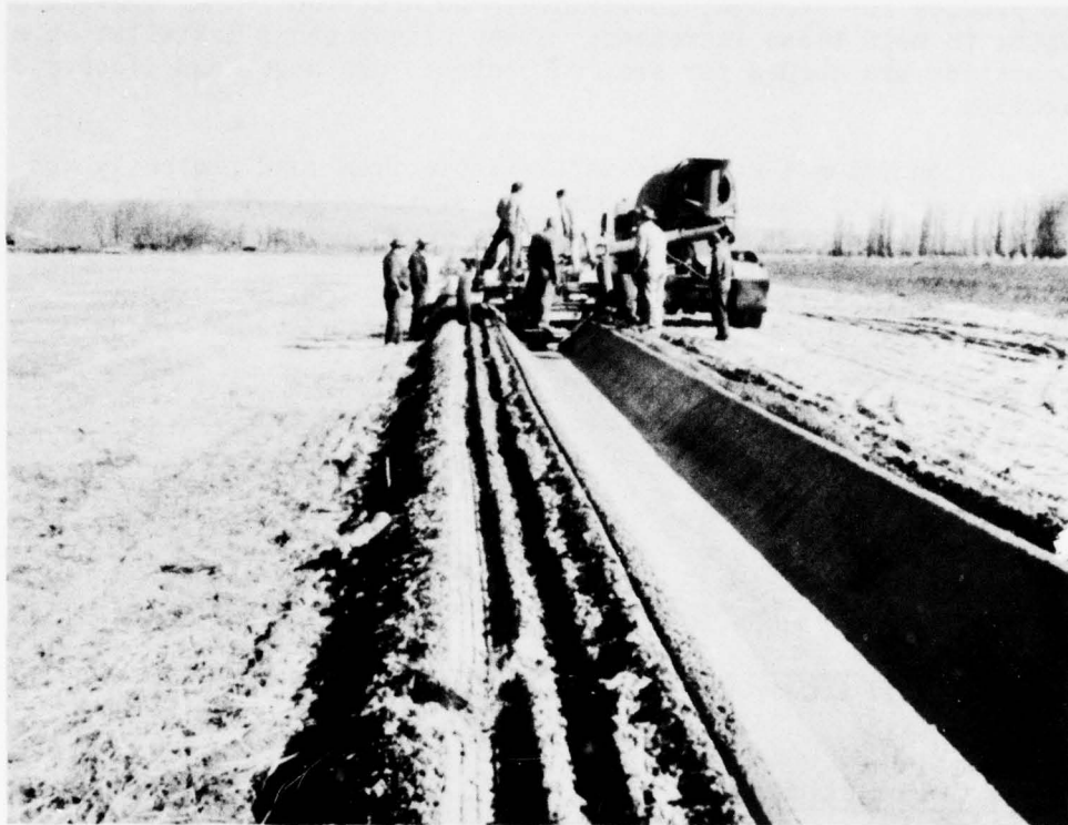
Concrete lined irrigation ditch to prevent water losses in transporting water to the fields. (SCS 0-1109-4)
