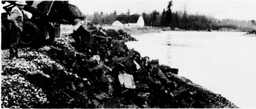
Rock riprap prevents bank erosion during high water flows. (SCS W-2210-10)
