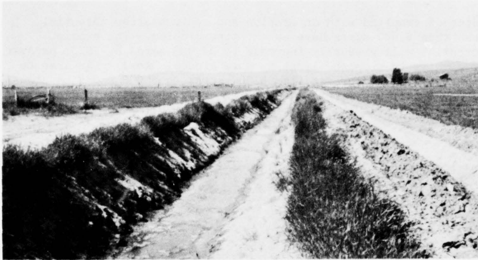
Surface and subsurface water disposal systems are essential in wet areas if cropland is to be seeded at the proper time and crops are to survive. Drainage also increases yields and reduces the cost of harvesting. (SCS 0-435-5)
