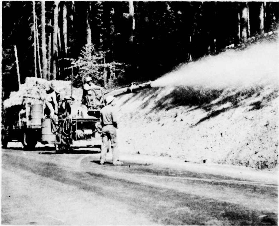
Hydro-seeder spreading a mixture of grass seed and mulch on a cutbank along a forest road in the subregion. (Forest Service)
