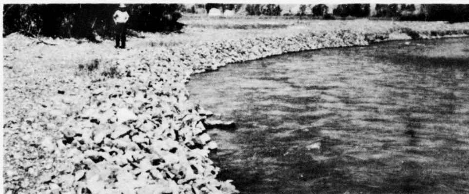
Stream channel diking and revetment prevent stream bank erosion and over bank flooding. (SCS F-137-17)
