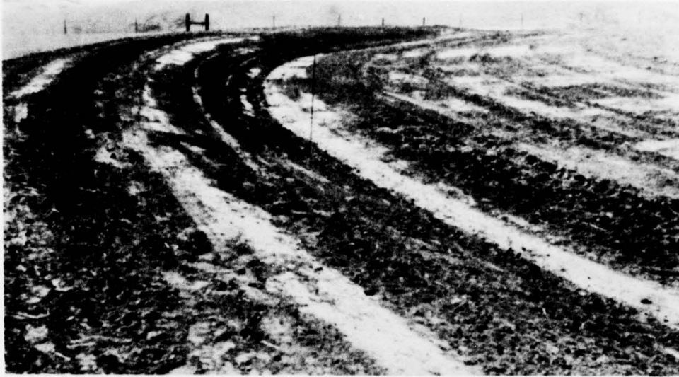
Diversion terraces control erosion while removing excess runoff. (SCS 0-1440-1)
