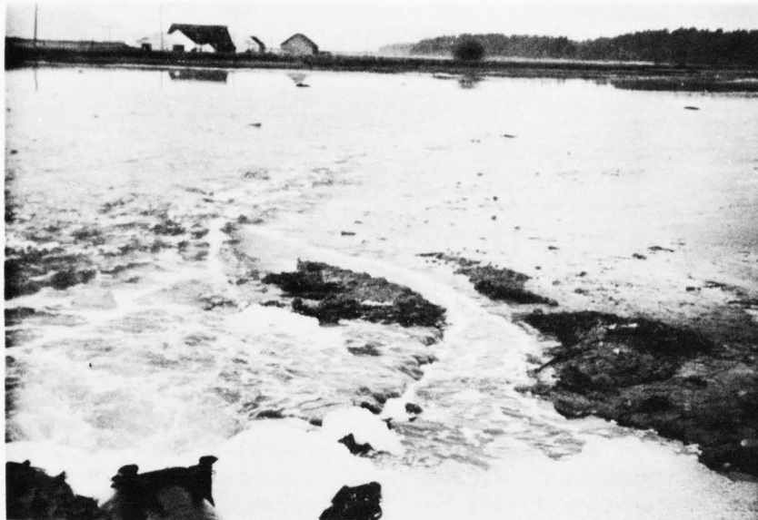
Flood gates prevent water from backing into lowland areas especially during high tide. (SCS W-1937-6)
