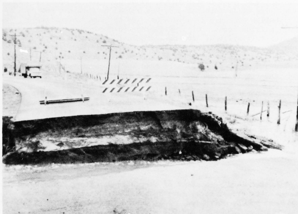
Road damage of this type disrupts traffic and requires additional maintenance and repair crews to keep the roads serviceable. (SCS 9-1698-9)
