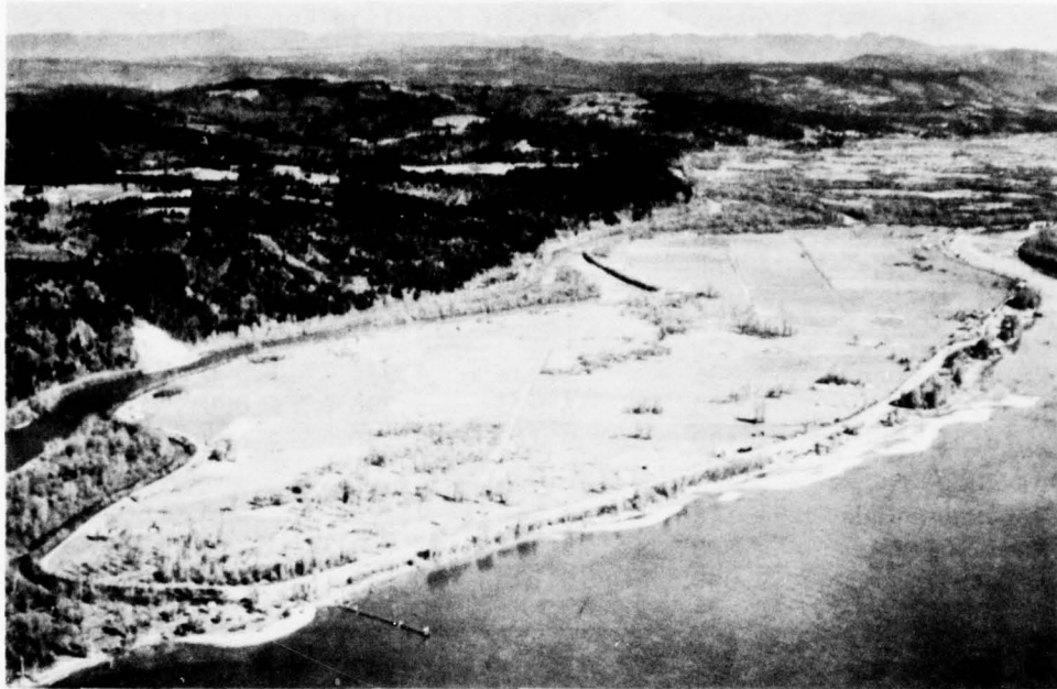
Drainage ditches and protective dikes are used extensively along the Columbia River. (SCS WN-8500-2)
