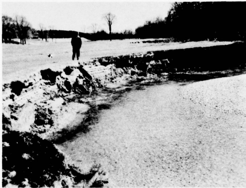
Stream undercuts the bank on the outside curve causing the bank to slough and slump into the river.
