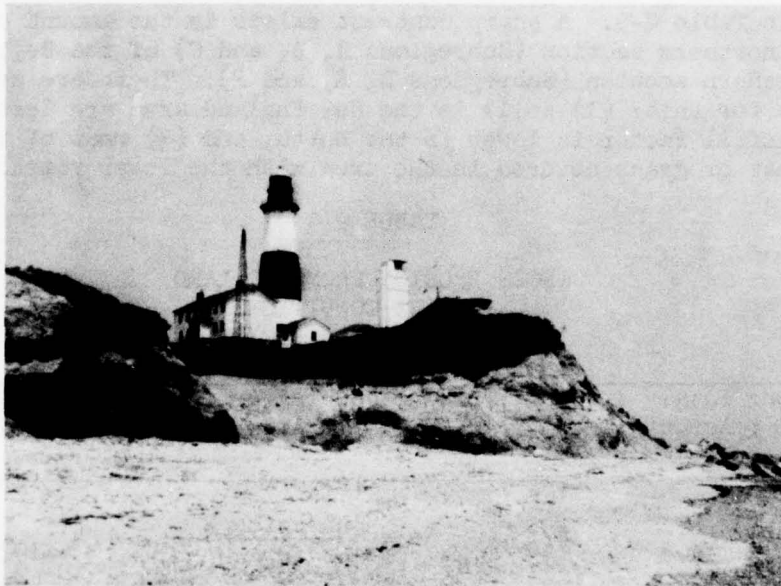
Lighthouse with eroding glacial till bluff is now several hundred feet closer to the edge.
