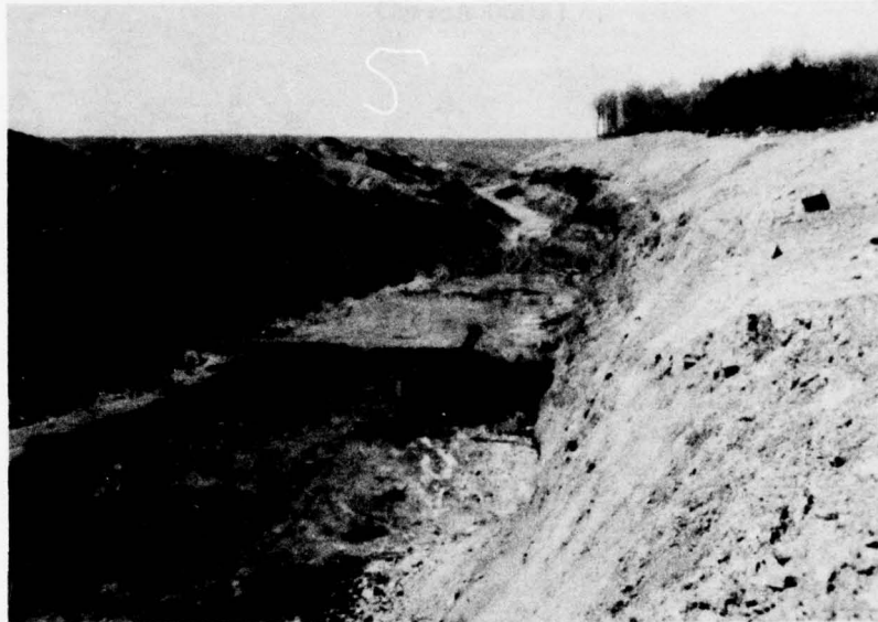
Fifty feet of overburden is being removed to expose coal seam in this strip mining operation.
