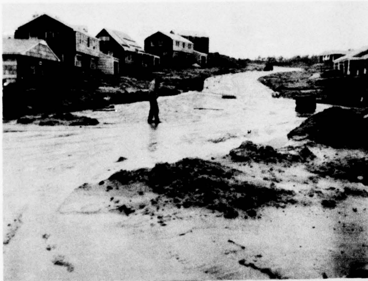
Excessive sediment is produced by an intense rainfall on exposed land.
