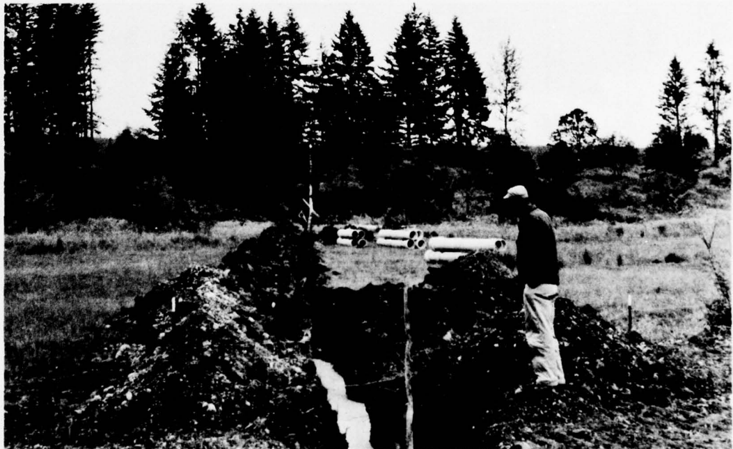
Photo III-2. A closed pipe irrigation system under construction. Efficient systems such as this will reduce distribution losses in the future. (U.S. Department of Agriculture Photo)
