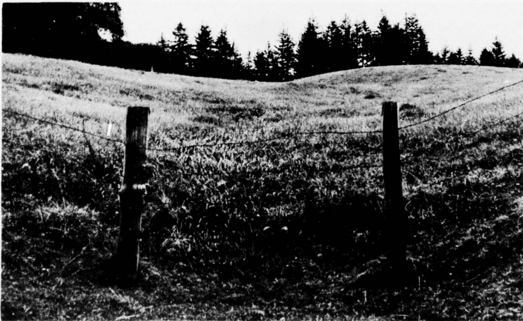
Photo II-14. A natural waterway is protected by a permanent grass cover, Subbasin 11, Clackamas County. (SCS Photo F-64-9)
