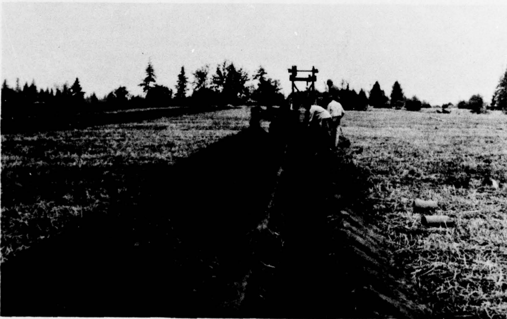
Photo II-29. Clay tile is laid in trenches in a pattern designed for good drainage near Gresham, Oregon. (SCS Photo 0-1049-7)
