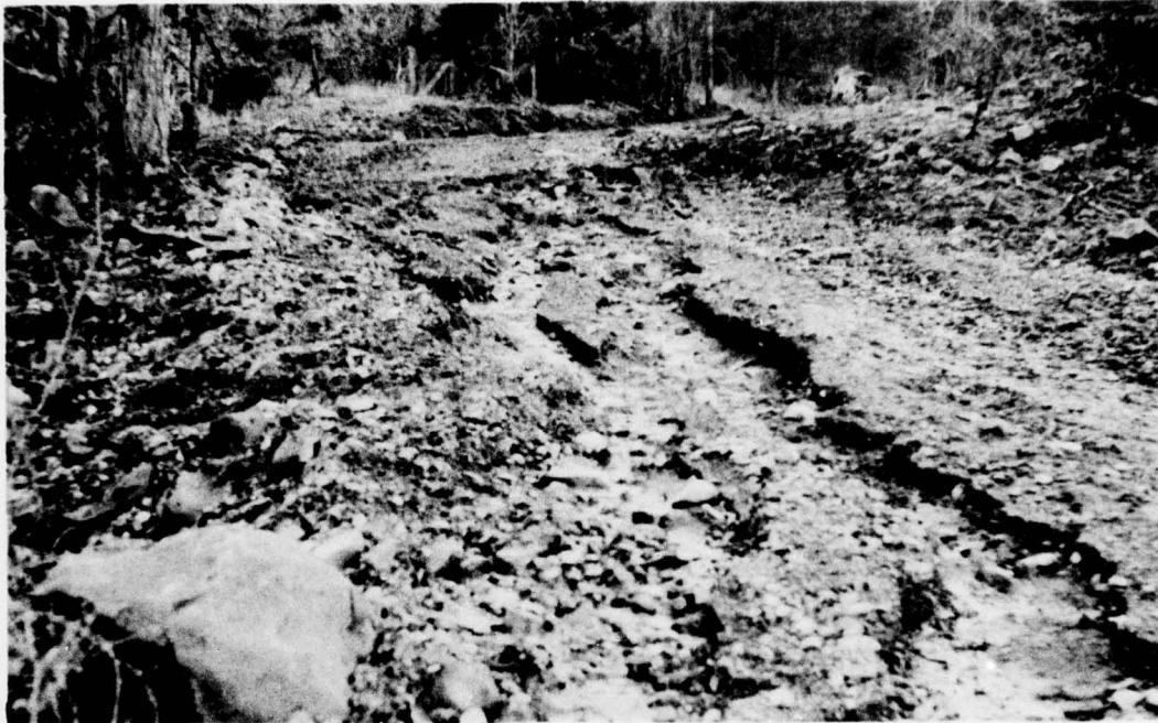
Photo II-40. Forest roads increase overland water flows and may cause erosion problems. (BLM Photo)
