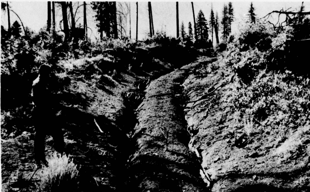
Photo II-38. Poor locations of skid trails and temporary logging roads plus inadequate drainage cause accelerated erosion. (U. S. Forest Service Photo 484291)
