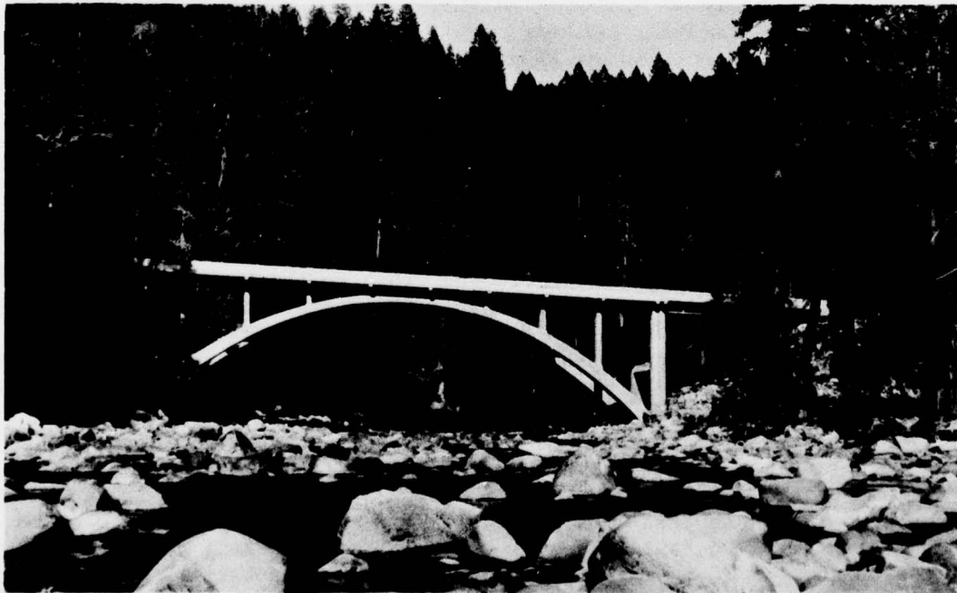
Photo III-9. A modern concrete arch bridge crosses the Collawash River and at the same time protects the water resource by allowing free fish passage underneath and no dumping of road waste in stream - Clackamas Subbasin. (U. S. F S Photo)
