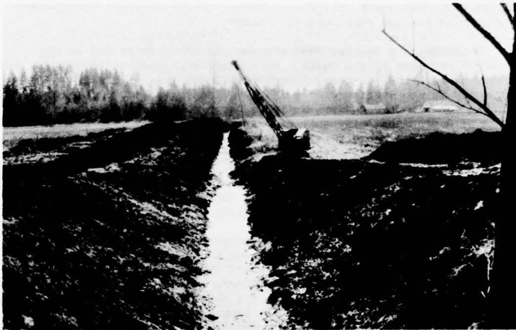
Photo I-3. Major drainage outlets are often necessary before on-farm drainage can function. Clackamas County near Butteville. (SCS Photo 0-1211-2)
