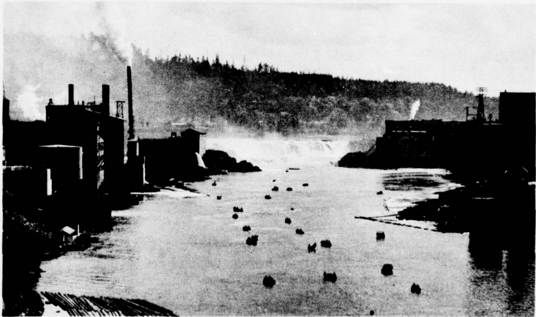
Photo II-17 Floating and suspended solids result from improper treatment of industrial wastes. (O.S.H.D. Photo)
