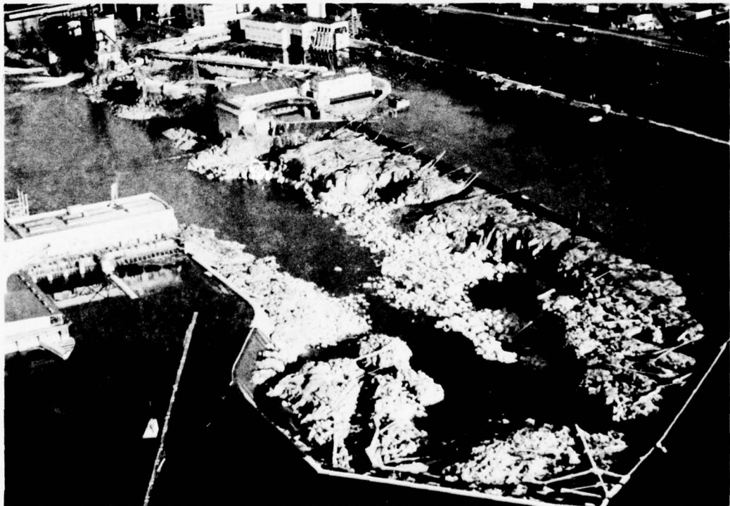
Photo II-7. Summertime low flow at Willamette Falls. Most of the river is being diverted through two power turbines.
