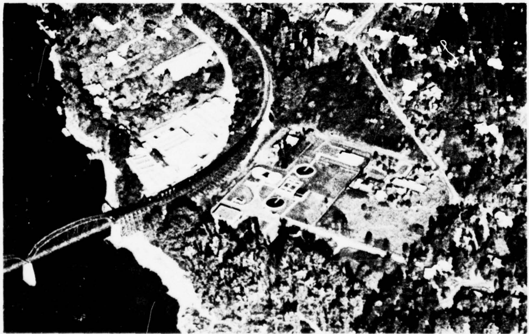
Photo IV-1. Two of the seven treatment plants in the Portland Service Area that discharge into the Willamette River: Lake Oswego (top) and Oak Grove.
