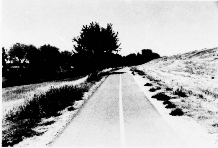
Photo 36. Bikeway between levee and small drainage ditch about midway in Woodlake area.
