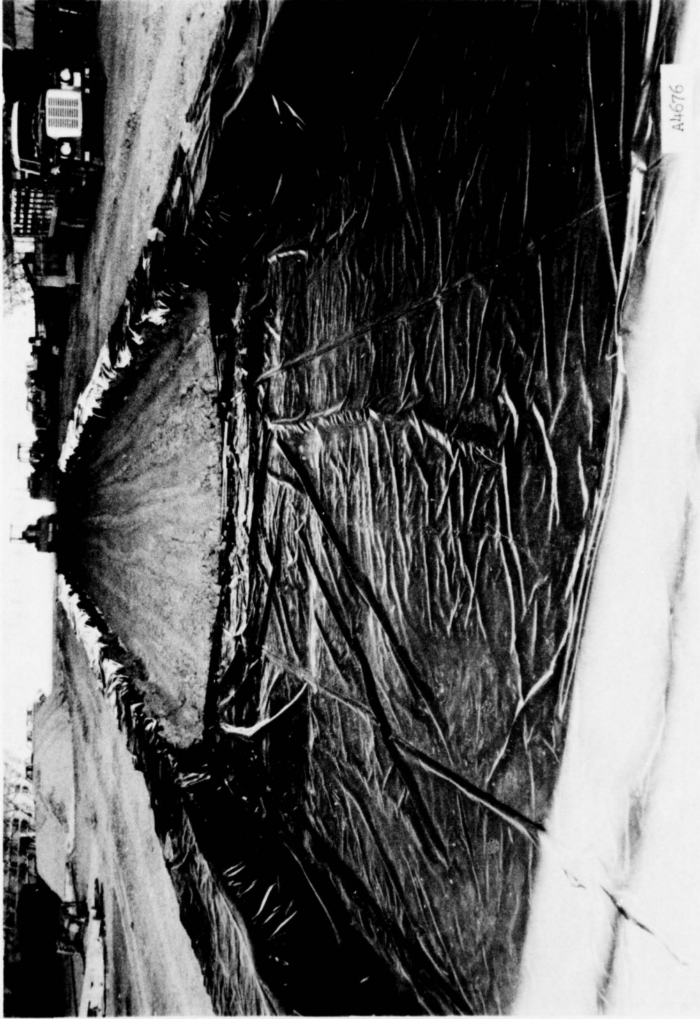
Photo 1. Installing soft clay subgrade on polyethylene
