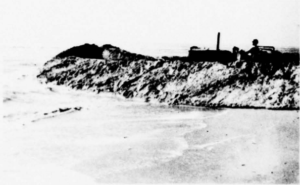
Building sand dike during initial excavation.
