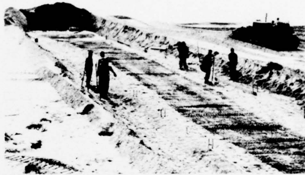
Grade prepared. Ready for hot sand-asphalt mix.
