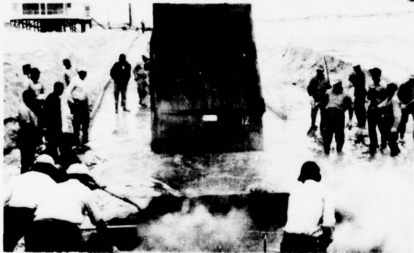
Apron and crown constructed in one operation. Crown shaped by hand.
