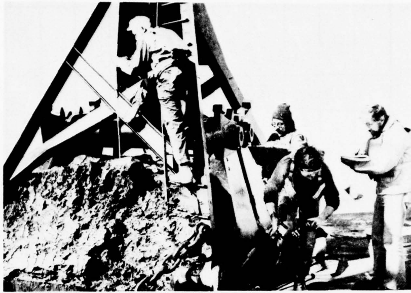
Figure 3-20. Dredged Material in the Clamshell
