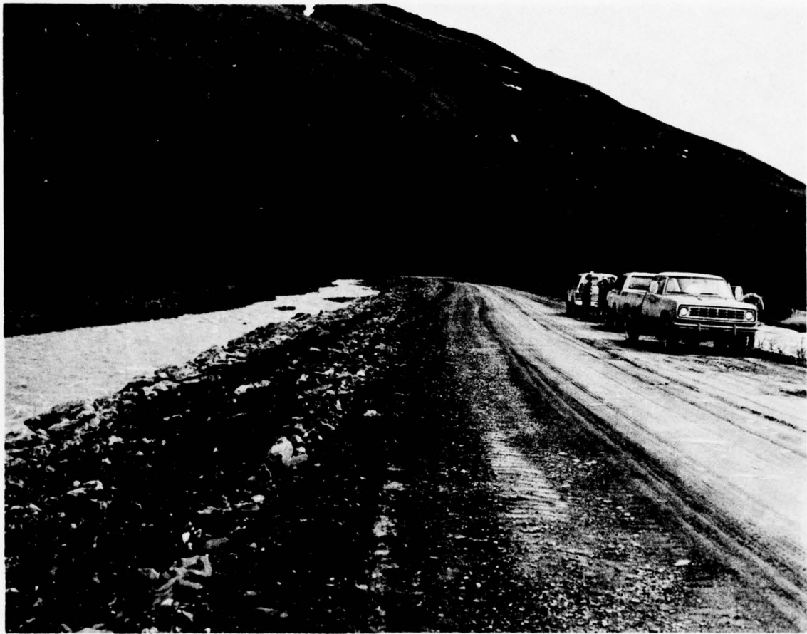
Figure 1. Channelization of the Dietrich River in the Brooks Range for the convenience of road and pipeline construction has led to accelerated bank erosion, stream siltation and excessive stream velocities, all of which have negative effects on fish spawning and migration.
