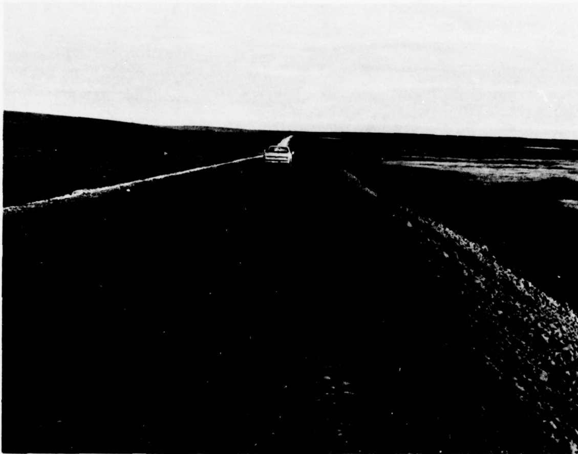
Figure 6. Oiling of the pipeline haul road to control road dust has resulted in the dispersal of oil, mixed with silt and water in road spray, onto the adjacent tundra downwind of the road as shown here. The consequences of the oil on the vegetation and the animals feeding on it are not known and should be the focus of investigations.
