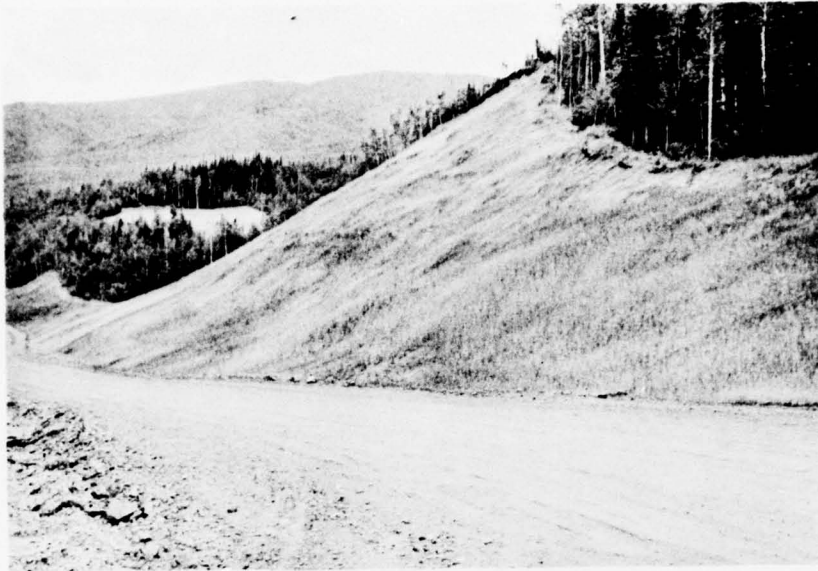
Plate 29. A.S. 51: Massive sandy slopes in vicinity of Rosa Creek. Hay and netting used to stabilize slopes as well as hydroseeded slopes in pipe storage yard and along access road.
