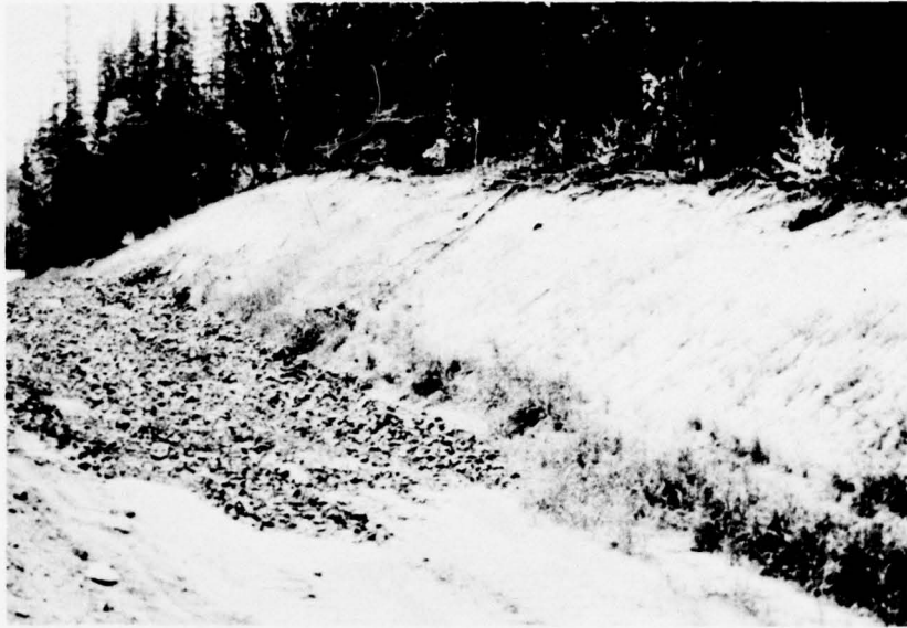
Plate 23. A.S. 80: Roadcut seeded on east side of Haul road north of 80-3.1. Germination very low on upper slope.
