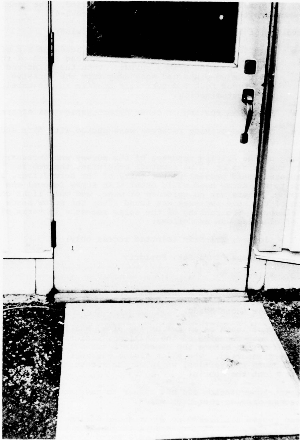
Figure B-3. Floor Panel Installation
