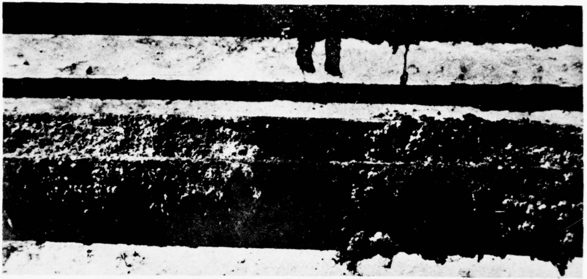
Figure A8. Typical fouling in the immersed zone.
