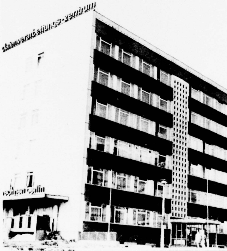
The Berlin VEB Maschinelles Rechnen Building is One of the Numerous Newly Built Data Processing Centers in the District Cities. Photo: Karin Kaiser
