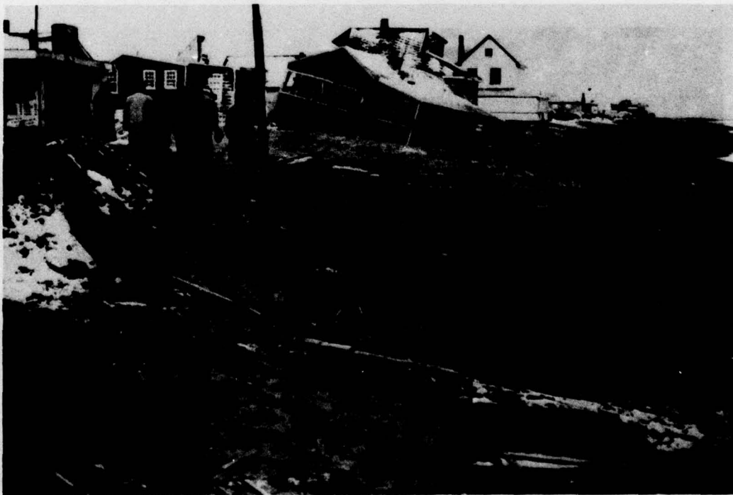
Figure 80. .Storm-damaged cottages at the northern end of Plum Island, February 1972.
