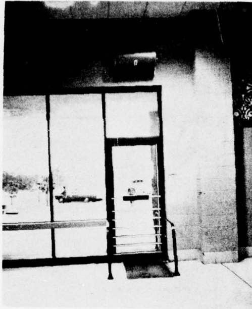
a. Air curtain machine installed 13 ft (3.96 m) above door and does not have an angle of throw of 15 degrees outward.
