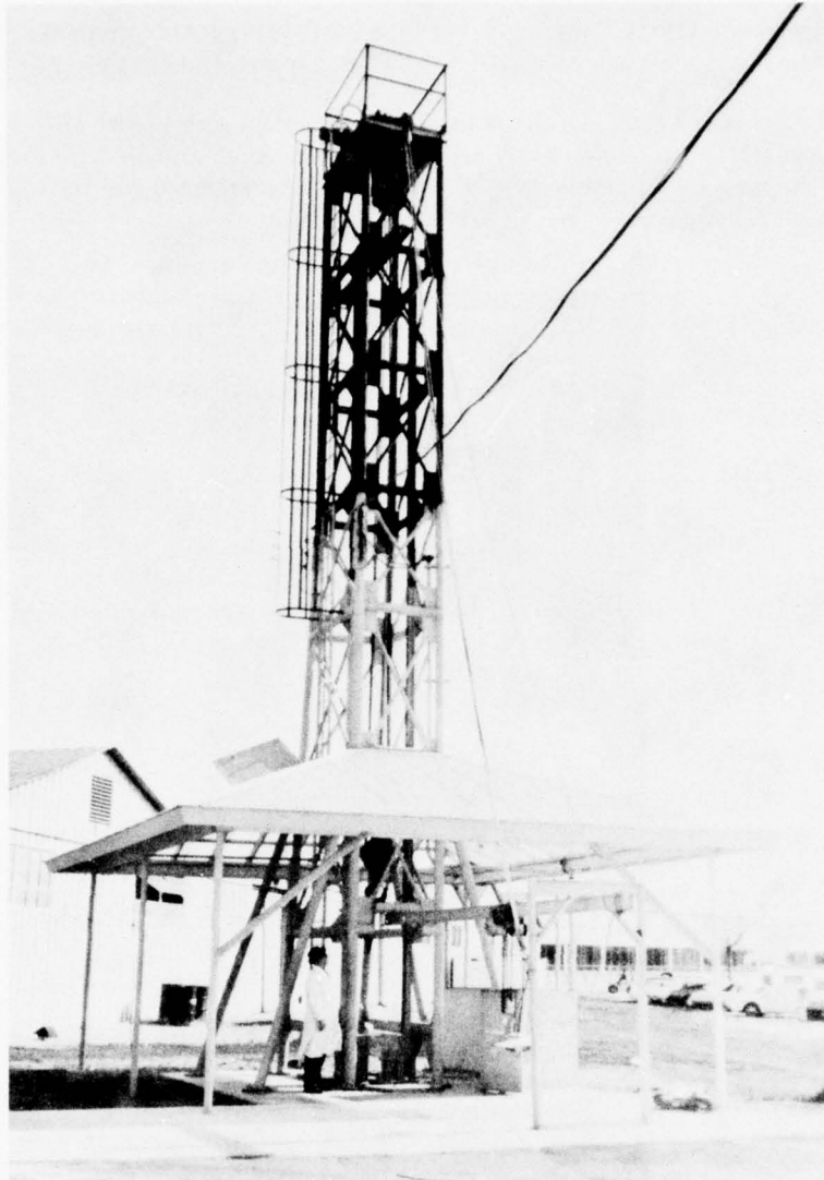
Fig. 107—DT test machine for 6- to 12-in. (150 to 300 mm) section sizes.
