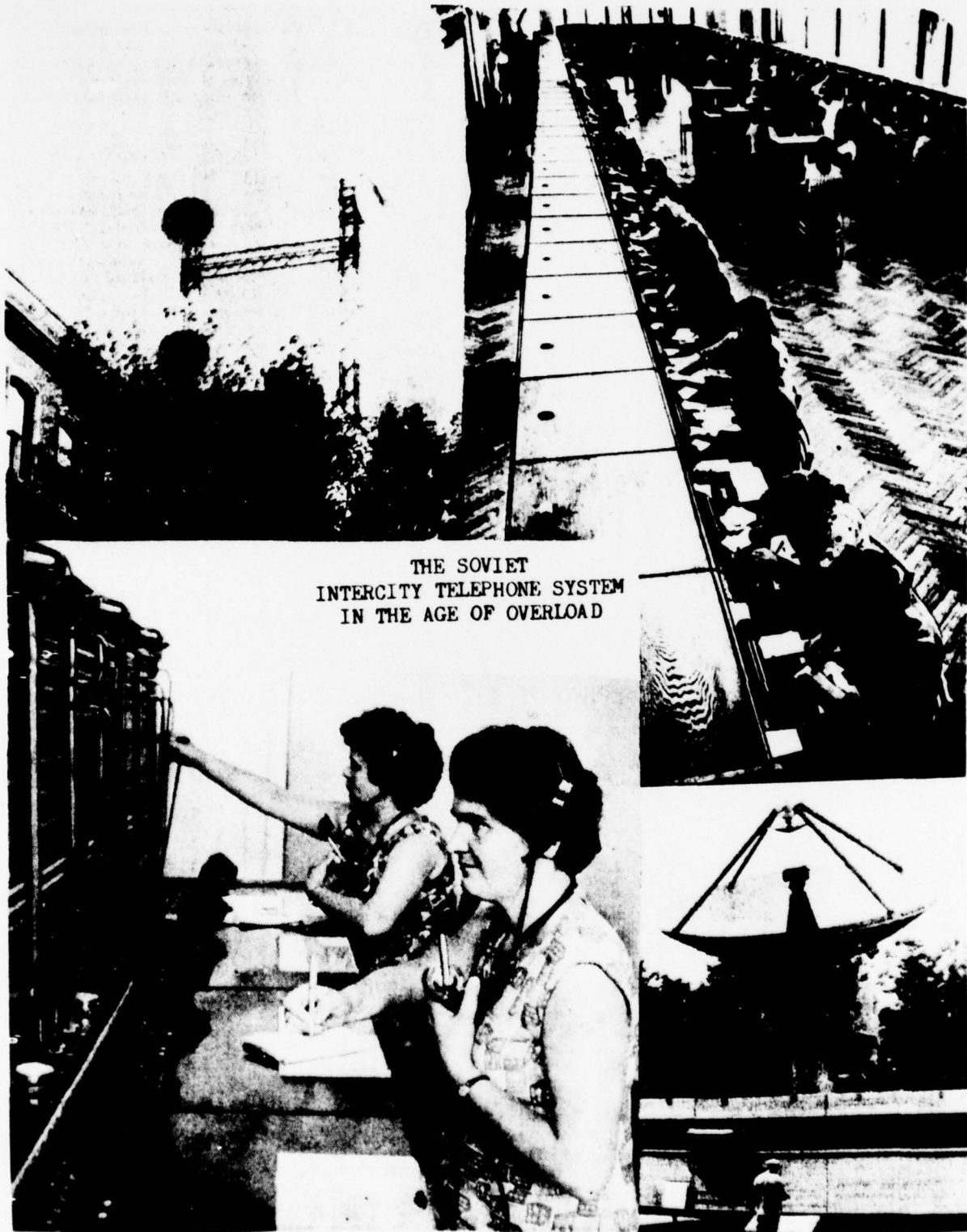
Figure a-1. Clockwise from lower left: M-60 switchboard ( Vestnik Sviasi No 9-1969 ); radio relay towers ( Tekhnika Molodezhi No 3-1976 ); Switchboard room of large intercity telephone station with M-60 switchboards ( Vestnik Sviasi No 1-1976 ); and probably "Mars" antenna ( Tekhnika Molodezhi No 3-1976 ).
