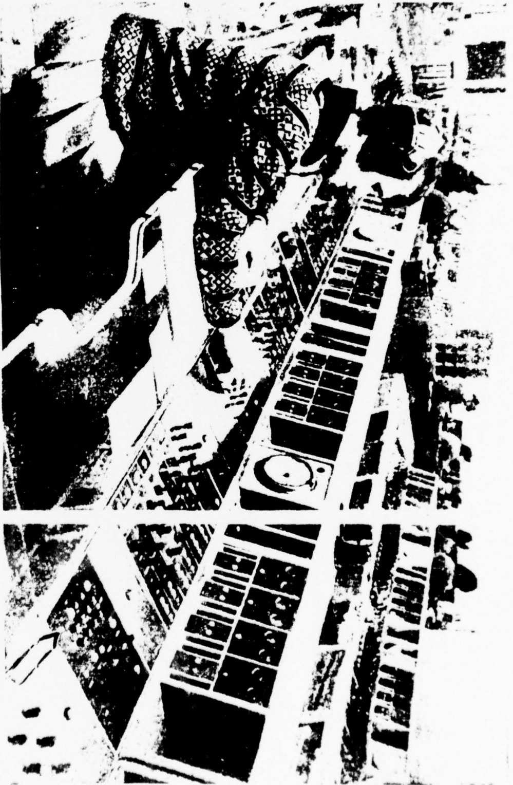
Figure J-1. AMTS-2 "cordless" intercity switchboard, which provides automatic distribution of subscriber calls among working positions, establishes order of priority of incoming calls (if no operator is available) and services delayed calls in order of appearance. Operators indicate readiness to receive calls by pressing a key. Eight digital lights have been installed on the front panel, on which number of subscriber making call, and his category, are automatically displayed. Note "touch tone" buttons (arrow) rather than dial. (Photo: Nauka 1 Zhizni No. 4-1970)
