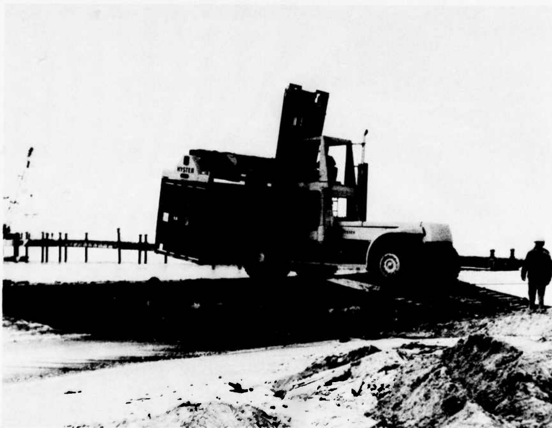
Figure 23. Top-lift loader removing 20-foot container from beached causeway during Lo/Ro test.
