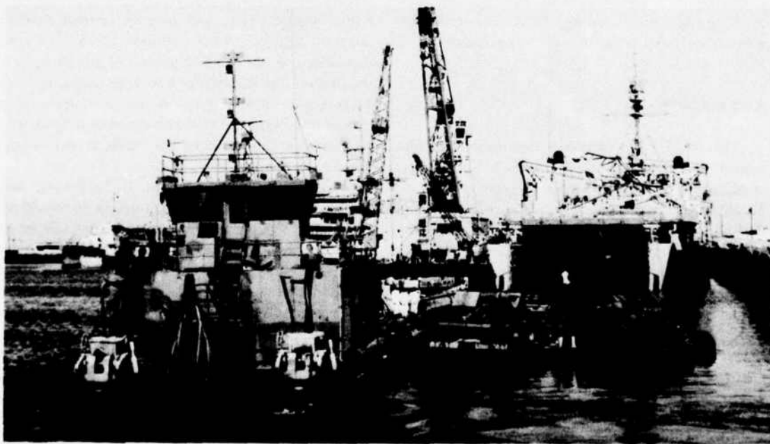
Figure 8. Loading elevated causeway components into LSD.
