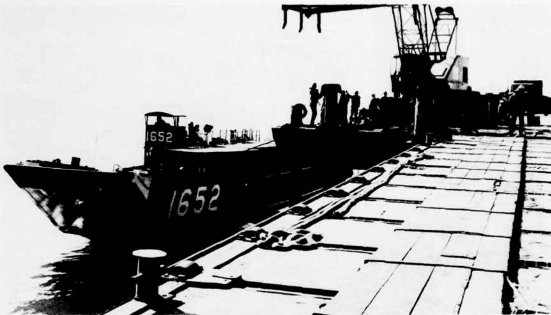
Figure 18. Class 1610 LCU, moored to elevated pier.
