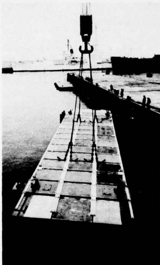
Figure 1. Causeway test section with internal and external spudwells.
