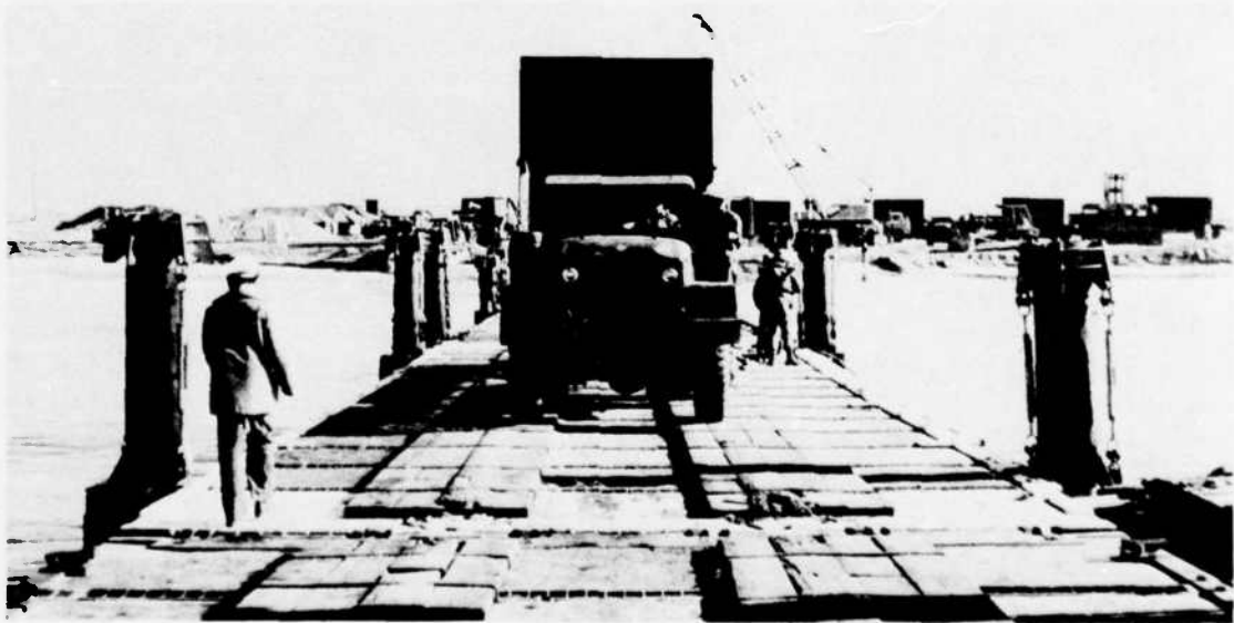
Figure 16. Pontoon deck reinforcement of 3x12 timbers provides roadway for vehicles.
