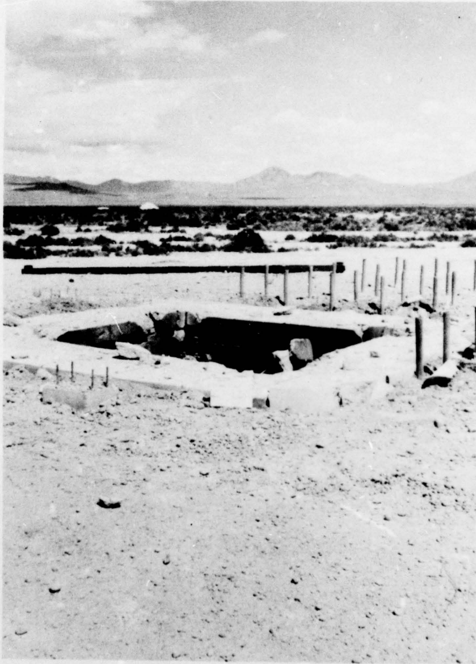
Fig 21 Post-test exterior view of Cell No. 1 (Test No. 7)
