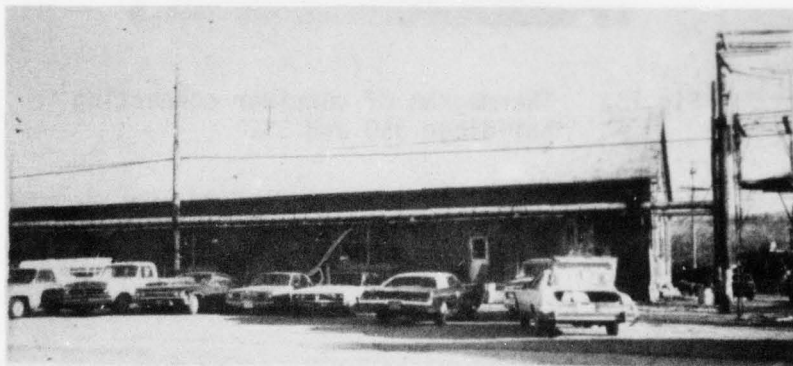
Fig 12b Photo of building 307
