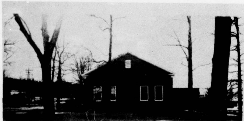
Fig 3b Photo of north end of building 183
