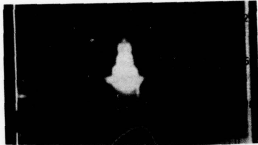
Fig 14a Thermogram of steam pipe and valve (Navy Hill)
