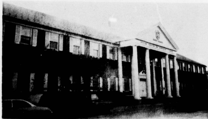
Fig 4b Photo of building 171
