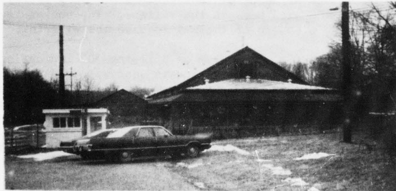
Fig 10b Photo of building 329
