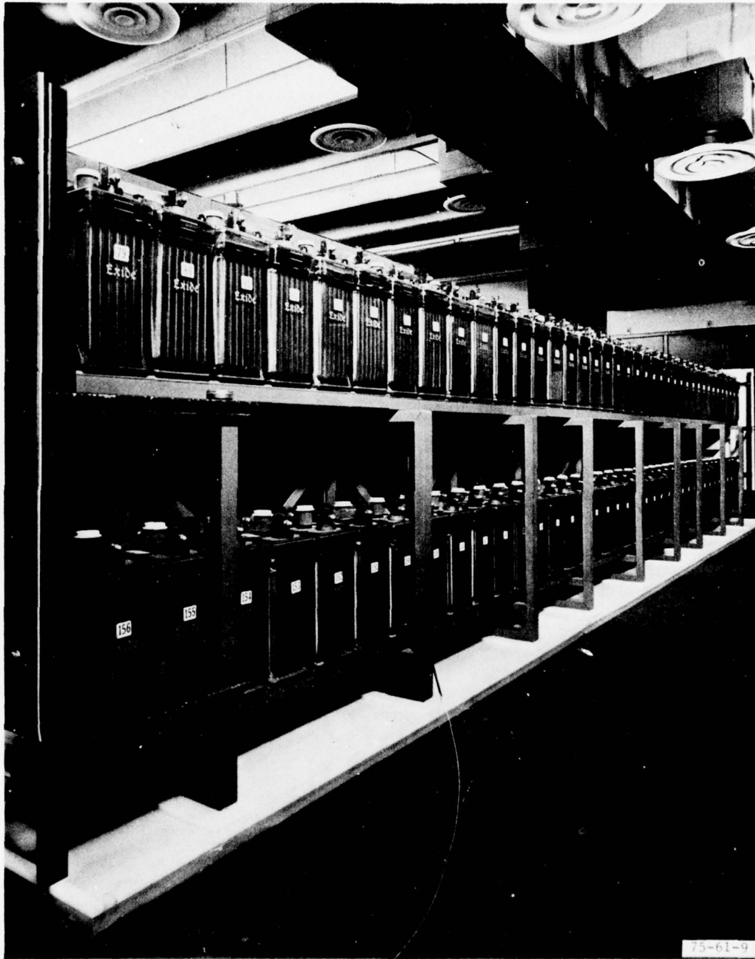
FIGURE 9. UPS LEAD-CALCIUM BATTERY CELLS
