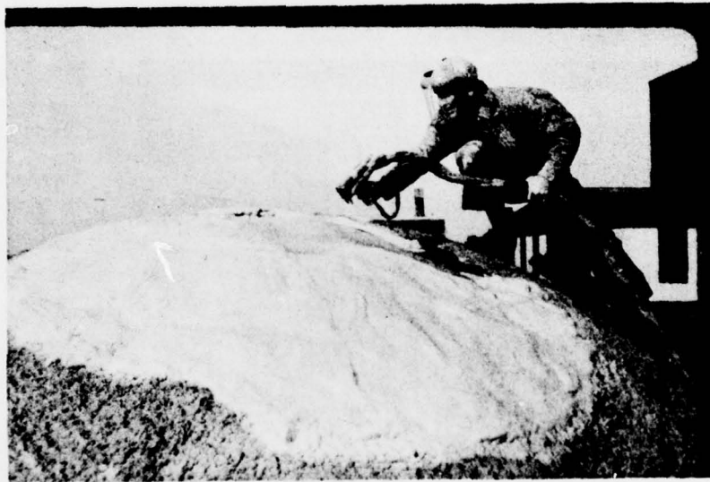
(b) Foam being applied to screen.
