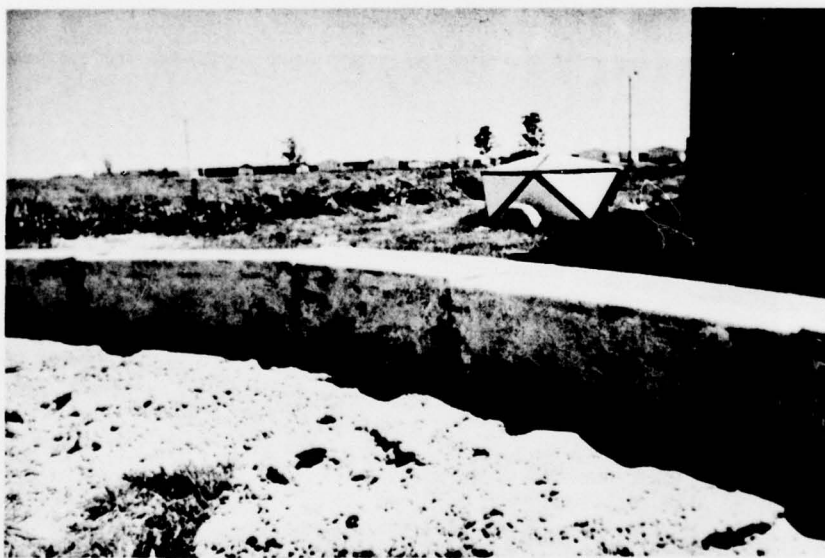
Figure 5. Segments of polyurethane foam/glass reinforced polyester ring beam for 28-ft (8.5-m)-diameter dome.
