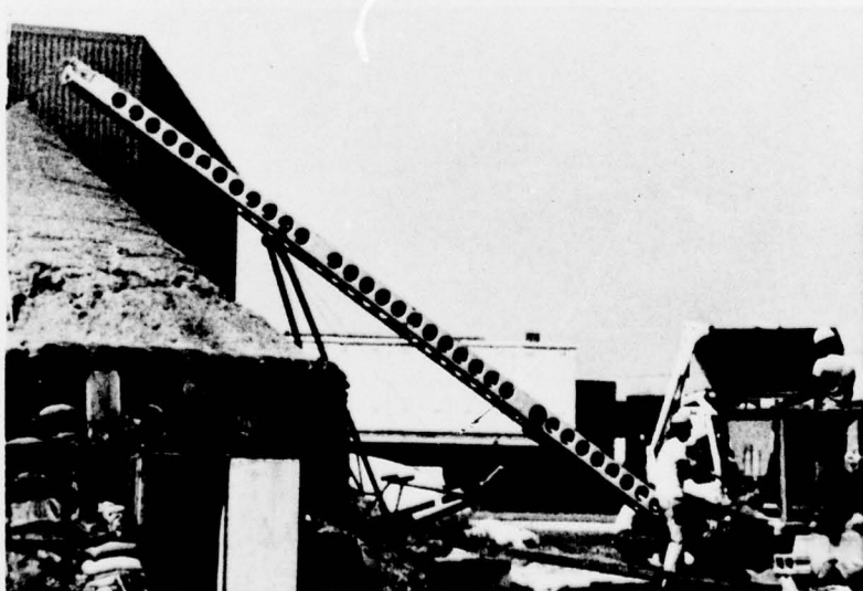
Figure 17. View of 18-ft (5.5-m)-diameter dome being loaded with 70 tons (63 503 kg) of sand to simulate a 4-ft (1.2-m) underground burial.
