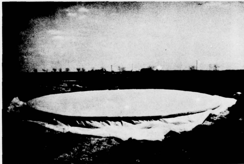
Figure 7(a). Lower membrane banded into position for 28-ft (8.5-m) dome.
