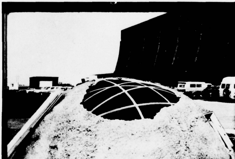
Figure 19. Deformed dome of Figure 15 being repaired using the foam/shotcrete system. This view shows the old material removed and flexible wood slats placed to curvature of dome.
