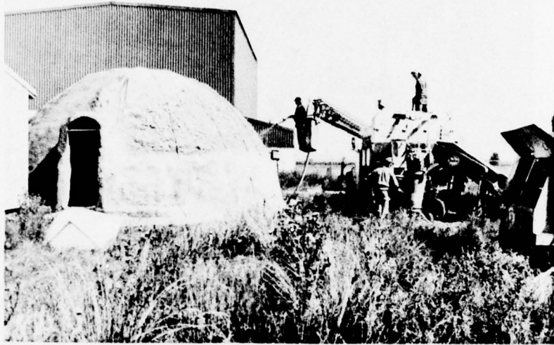
Figure 18. Batching of steel fiber concrete mix. Equipment required is a concrete mobile, a shotcrete machine, 600 cu ft (17 m 3 ) /min air compressor, and a truck-mounted snorkel crane.
