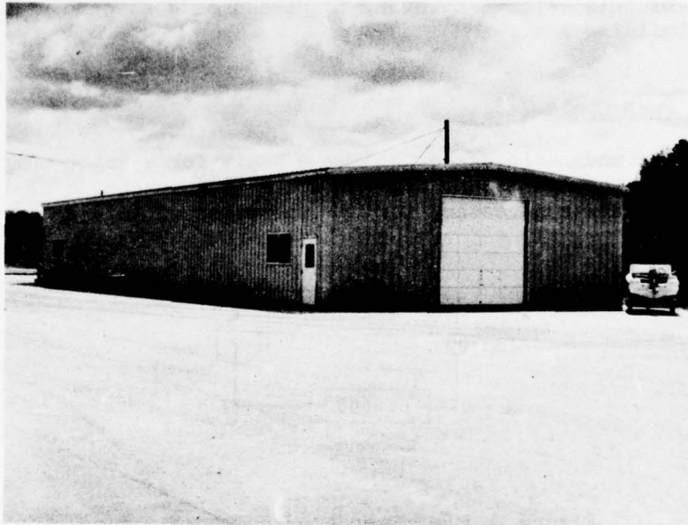
Figure 1. Equipment storage and fabrication building, 40 ft (12.2 m) x 100 ft (30.5 m) x 14 ft (4.3 m).
