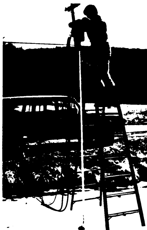
FIGURE 18. Driving a 10-ft-long, 1-1/4-in.-OD electrical conduit through the lake ice cover into the bottom sediments using the Hydraulic Stake Driver-Retriever II.
