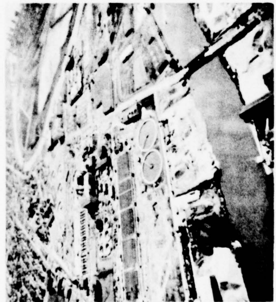
Construction at Jefferson Avenue treatment plant in Detroit
